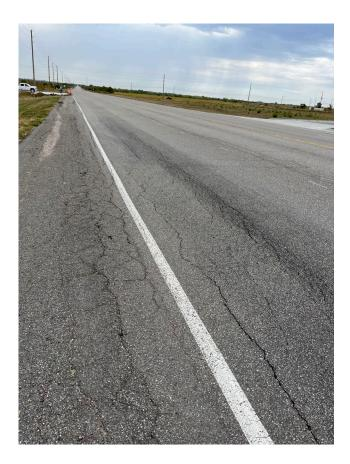
As mentioned above, the shoulder of Webb Road was initially constructed of 2" of asphalt onto a compacted dirt base. This combination is enough for an occasional use, but not for continued use of heavy construction traffic. The repaired/replaced section will consist of a 6" crushed concrete base and 6" of asphalt. The crushed concrete base will extend 1' beyond the surface asphalt to provide additional stability for the asphalt surface.
