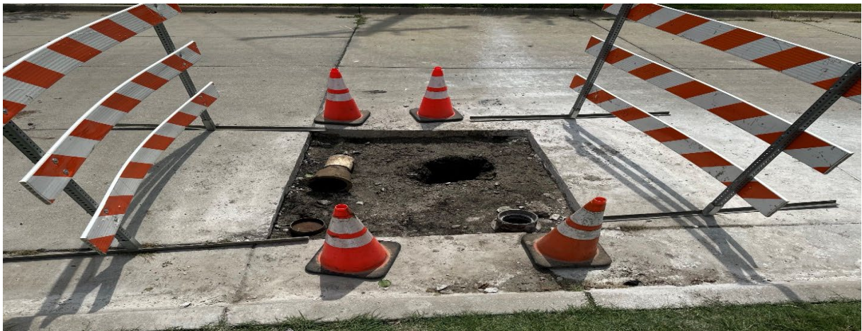
48 th and Hedgerow concrete removal to allow us to get on the 12" Valve
