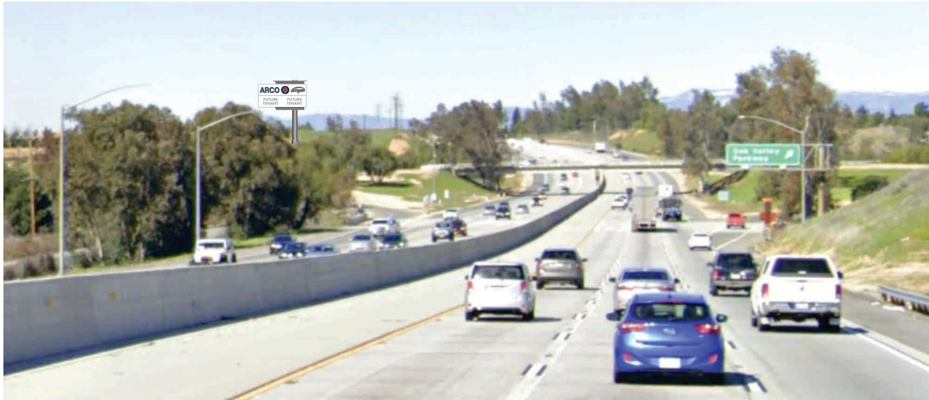
10 Freeway Traveling West approaching Exit 92
