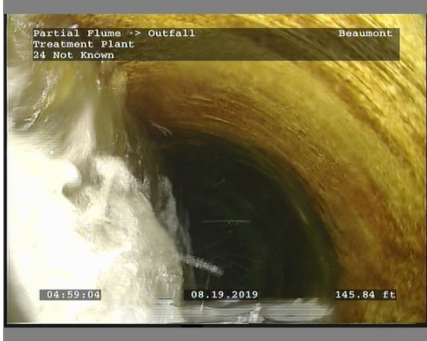
Photo: Partial Flume-Outfall-8192019-145.8386-050003.JPG 145.84FT, Camera Underwater, Finish
