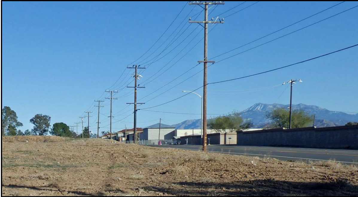
Figure 11. Transmission Line along First Street, towards California Avenue, Beaumont (ESE).
