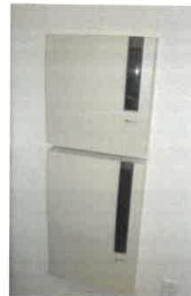
FTTH internet modem in closet of homes in Beaumont's Fairway Canyon served by Greenfield Communications
