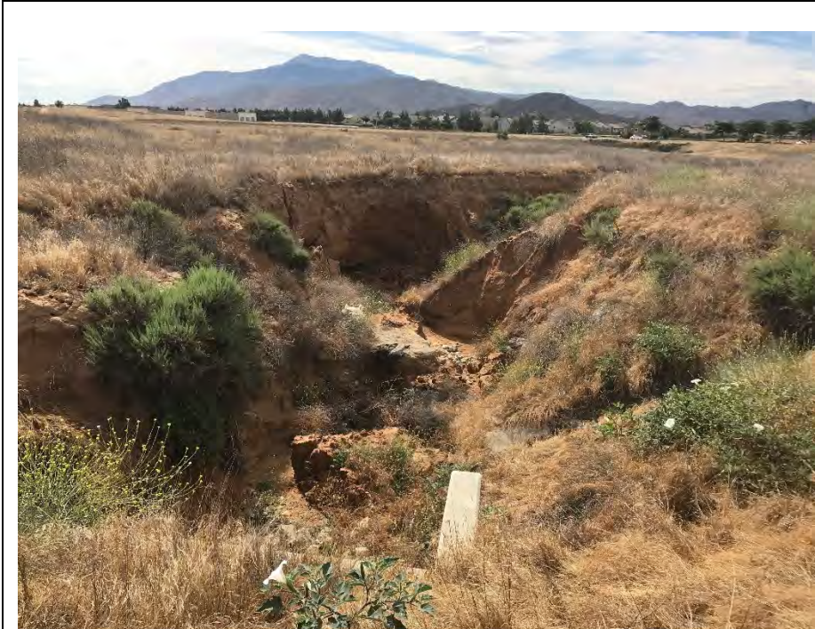
Photo 5 – Drainage B canyon connected to box culvert.
