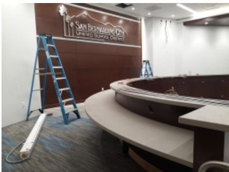
SBCUSD Board of Education (In Progress) San Bernardino, CA
