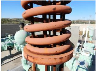
Corrosion at CAVs (typical)
