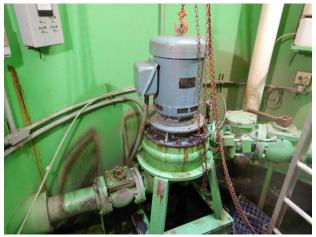
Pump #2, leak at pump/motor
