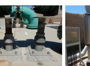
Cracking at pipe support concrete bases (typical)
