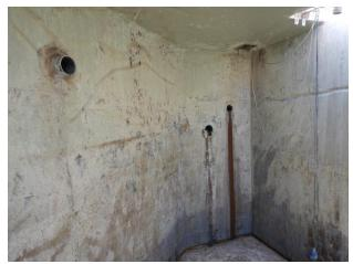
Corrosion staining on southwest wall
