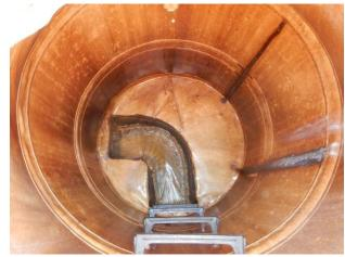
Bypass MH interior, pinholes in liner
