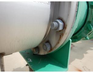
Dissimilar metal bolts/nuts used on SST pipe
