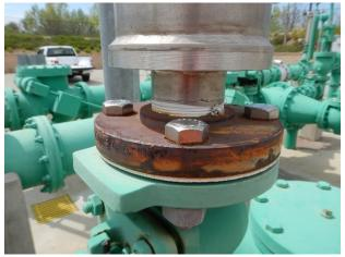
Corrosion typical at bolts/flanges due to contact between dissimilar metals (including SST)
