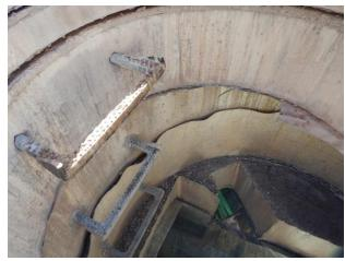
Liner disbonding from the concrete
