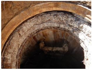
Non-mortared joints with exposed aggregate
