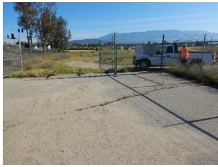
Cracking in asphalt near entrance
