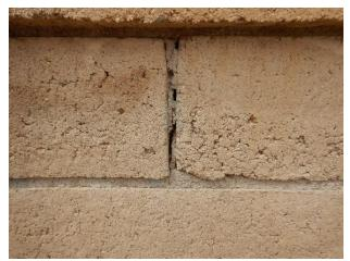
Mortared joints cracked with voids (typical)
