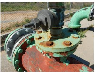
Surface corrosion (closeup)
