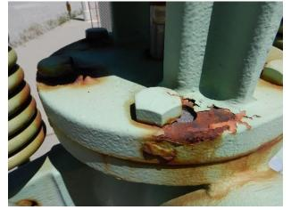
Corrosion typical where coating has flaked
