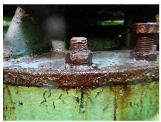
Pump #2 corrosion due to leak (closeup)
