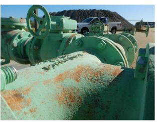
Surface corrosion typical throughout piping
