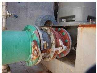
Corrosion typical at SST flanges and tie rods, dissimilar metals
