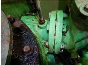
Pump #2 corrosion at bolts/flanges
