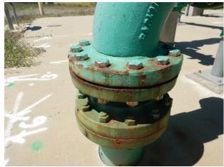
Corrosion typical at bolts/flanges (likely due to dissimilar metals)
