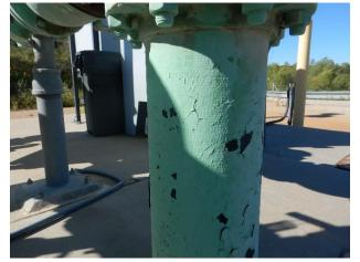
Coating peeling/flaking at riser sections (typical)
