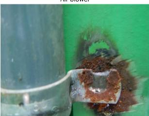
Corroded hardware at conduit supports
