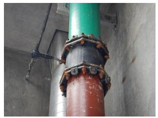
Corrosion typical on hardware at flexible couplings
