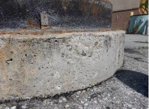
Exposed aggregate at wet well concrete collar
