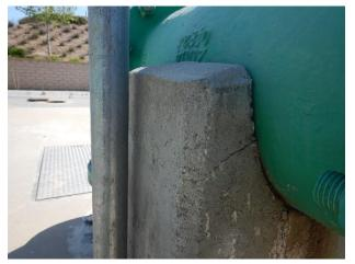
Cracking under Pump #2 pipe support
