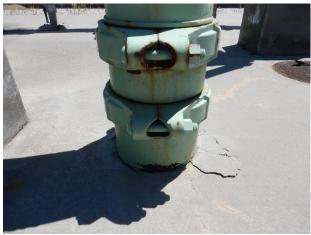
Crack in concrete at Pump 1 discharge header
