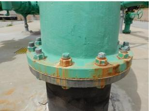
Corrosion typical at bolts/flanges
