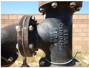
Minimal surface corrosion typical at flanges
