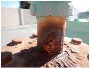
Corrosion at ARV tap connection (Pump 1)
