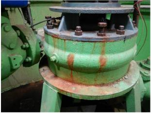
Pump #1 corrosion at bolts
