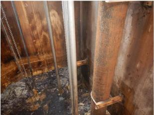
Surface corrosion typical throughout pump discharge piping
