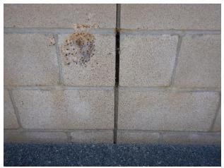
Spalling pocket on interior of south CMU wall
