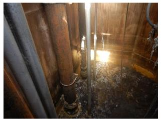
Surface corrosion typical throughout pump discharge piping
