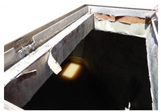
Liner disbonding at top of the structure
