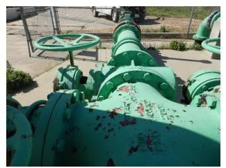
Cracked/peeling coating with corrosion typical throughout piping
