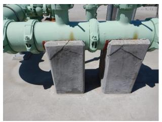
Cracked concrete pipe supports at Pump #3 ARVs; pipe shifted to left in photo
