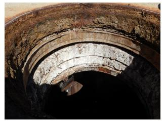
Bypass MH exterior, corrosion at rim
