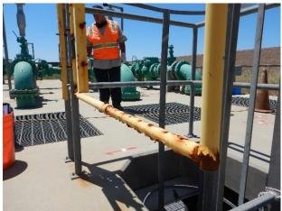
Dry well access swing gate corroded throughout
