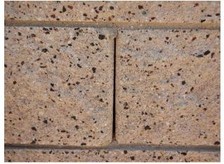
Missing mortar at vertical CMU joints (typical)
