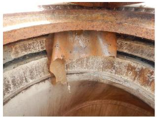
Bypass MH rim, remnants of plastic film, unmortared joints
