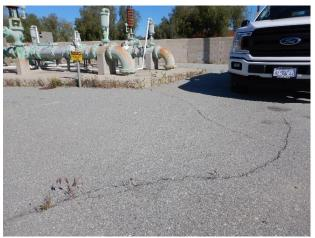
Cracked concrete base at pipe supports spanning Crack in asphalt spanning from wet well structure towards the entrance gate (0.2")
