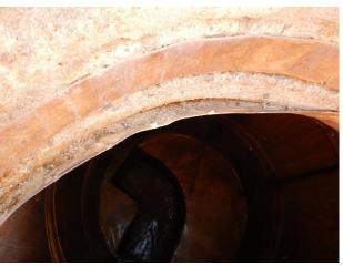
Bypass MH liner disbonding from cone
