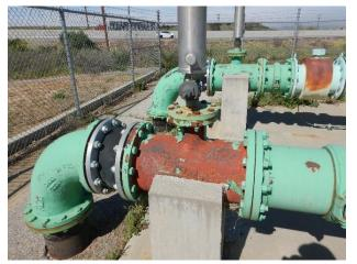
Surface corrosion typical throughout piping
