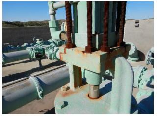
Corrosion at CAVs (typical)
