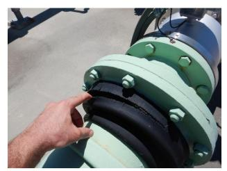
Cracking external rubber seals (typical)
