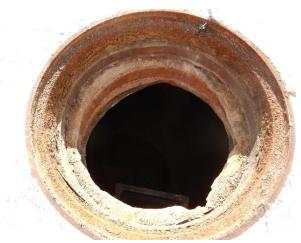
Bypass MH exterior, corrosion at rim
