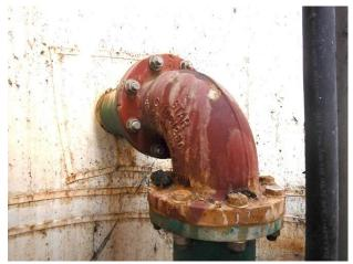
Pump discharge piping, minor corrosion at bolts/flanges
