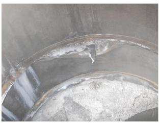
Liner disbonding from concrete (typical)
