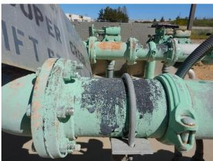
Factory coating evident through thinned coating (typical)
