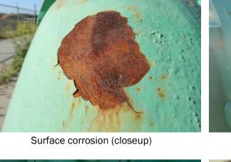
Surface corrosion typical throughout piping
