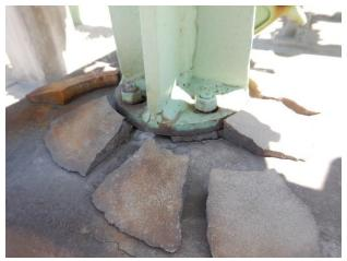
Cracked concrete collar at 4-in flange-mounted pipe support (typical)
