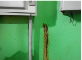
Corrosion where lined has failed (NW wall)
