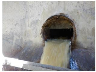
Influent pipe, heavy corrosion (closeup)
