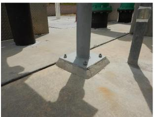
Concrete base for metallic pipe supports
