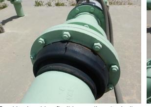
Cracking in rubber flexible couplings (typical)
