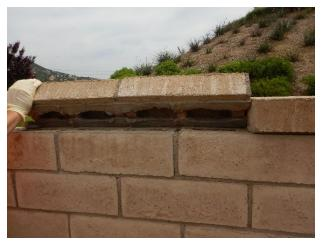
Masonry wall cap loose
