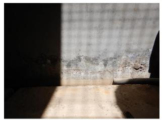
Spalling typical at 0" – 16" AFF, east wall
