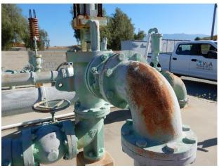
Surface corrosion typical throughout piping
