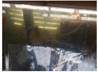
Sump pumps submerged, corroded
