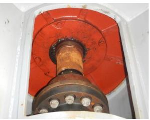
Corrosion on pump shaft (Pump 4)
