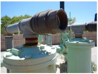
Corrosion at ARV threaded connections (typical)
