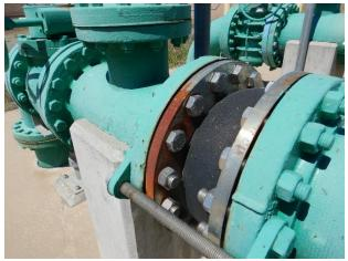
Corrosion typical where there is contact between dissimilar metals
