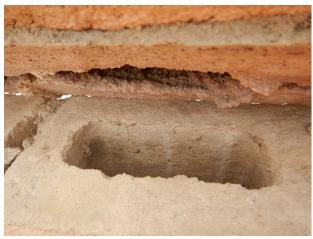
Missing grout inside of south wall
