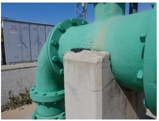
Cracking under Pump #1 pipe support
