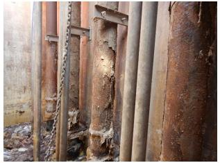
Heavy corrosion on pump discharge piping (VANDA 4; typical)
