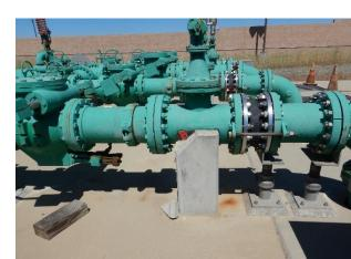
Cracked concrete pipe support (Pump 1)
