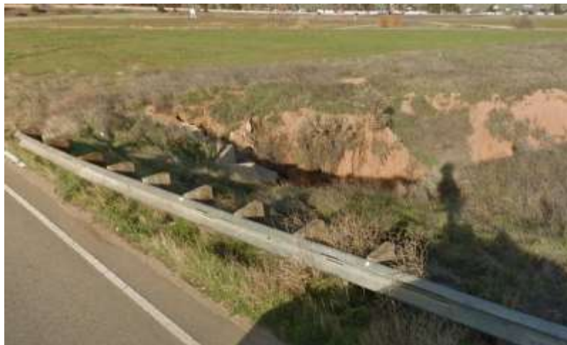
Figure 9. Existing Culvert due East of Pennsylvania Avenue.
