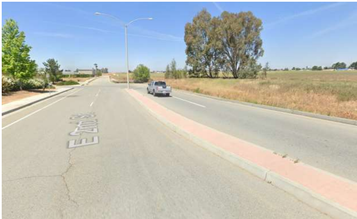
Figure 21. 2 nd St., A Divided Collector Due West.
