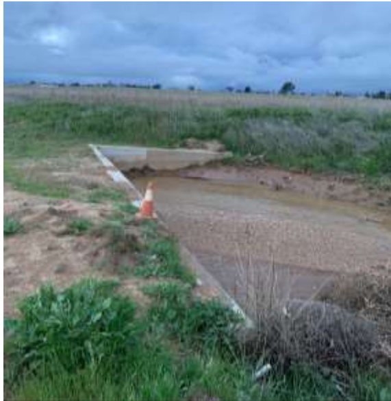
Figure 7. Existing Culvert/Storm Drain South of E. 2 nd St.
