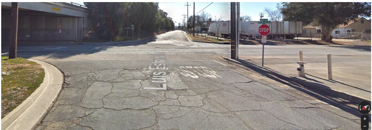
Figure 7 - Existing Traffic Control Devices and Striping at Eastbound Luis Estrada Road
