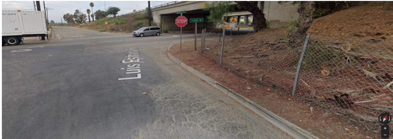
Figure 8 - Existing Traffic Control Devices and Striping at Westbound Luis Estrada Road
