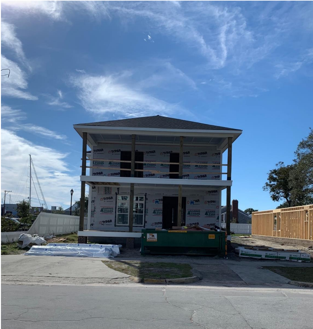
312 Ann Street – Current house/construction
