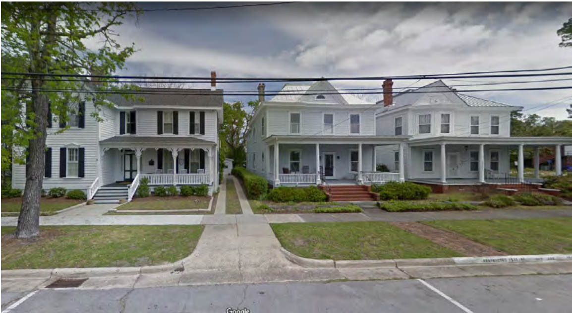
Street view East on Ann Street
