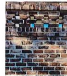
Brick Foundation General Shale - Silas Lucas
