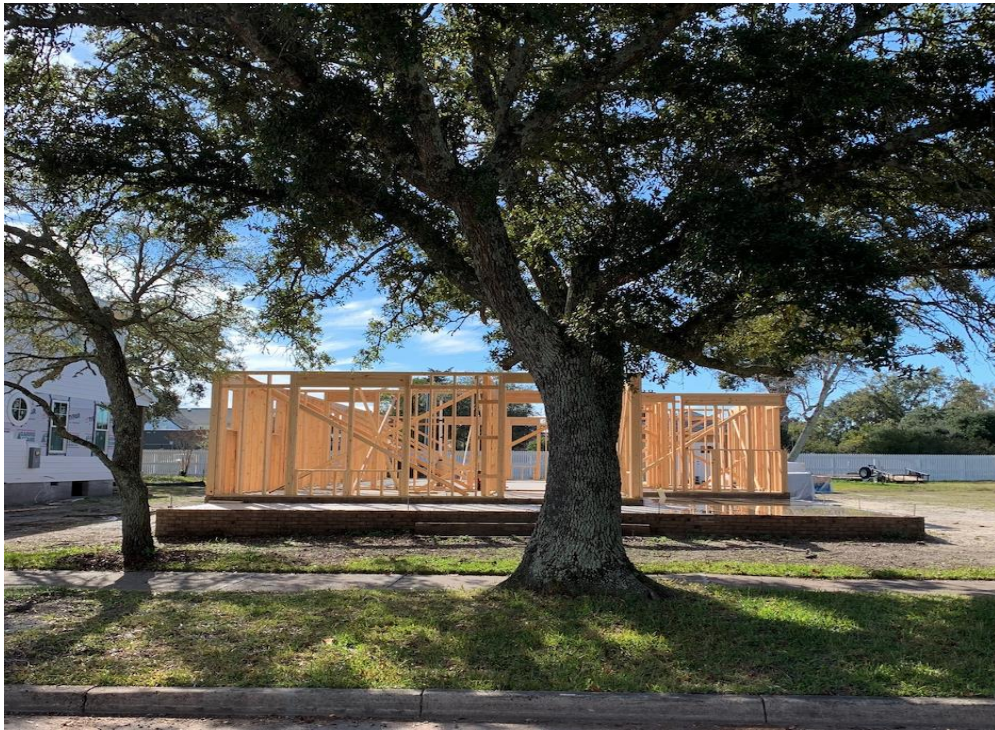
310 Ann Street (directly next door to 312 Ann Street - House under construction)
