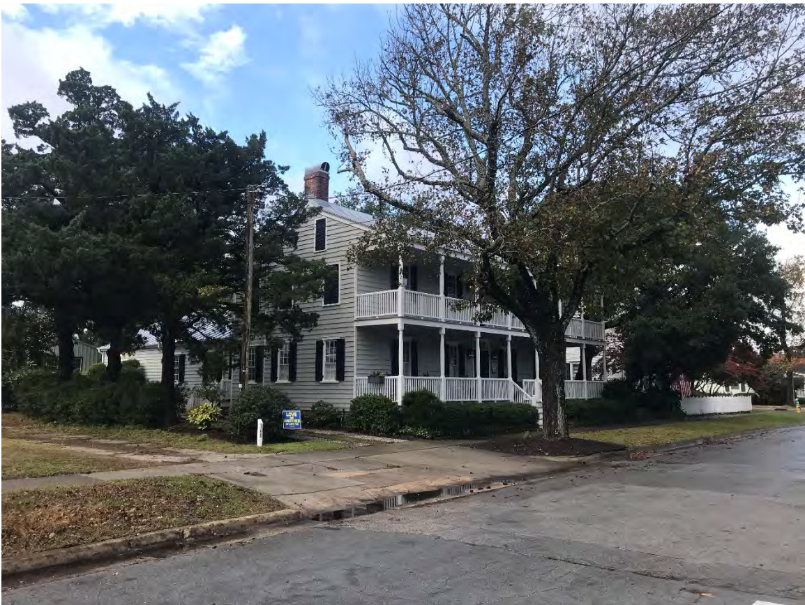
Street view West on Ann Street
