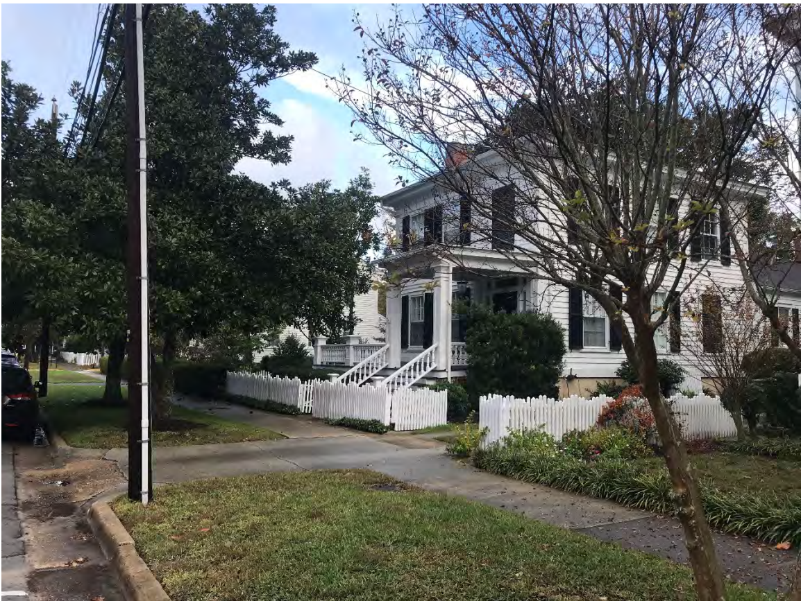
Street view West on Ann Street
