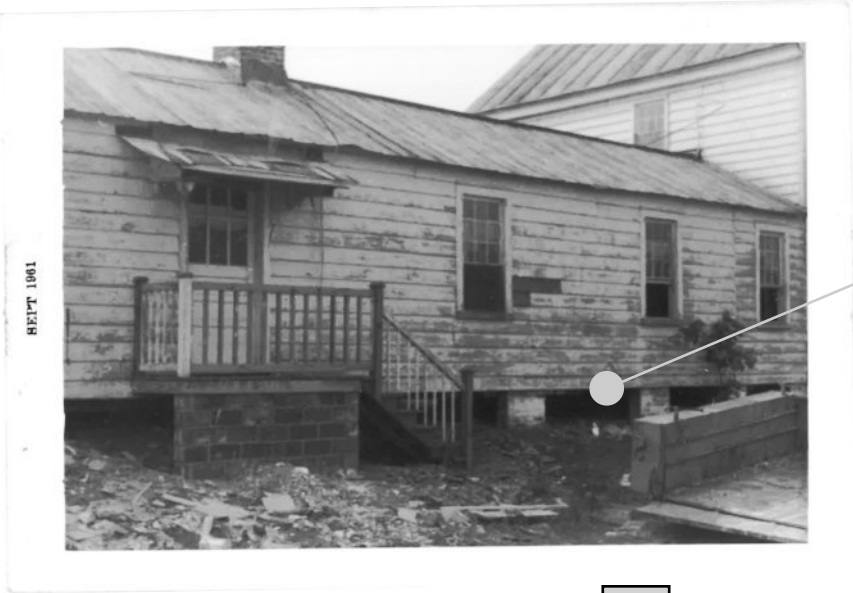
Area where foundation screens to be replaced between brick piers
