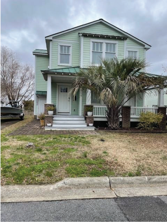
309 Moore Street (across Moore Street)
