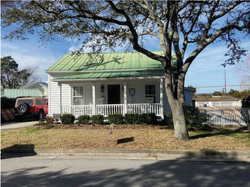
305 Moore Street (across Moore Street)
