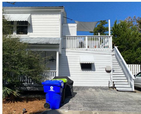
SOUTHEAST CORNER TAKEN FROM DRIVEWAY
