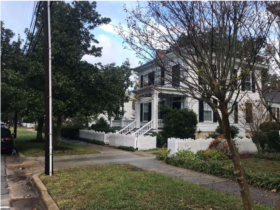
Street view West on Ann Street
