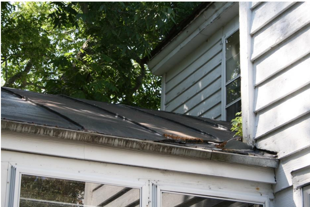
Rear view of 302 Cedar Street (proposed location for new addition)
