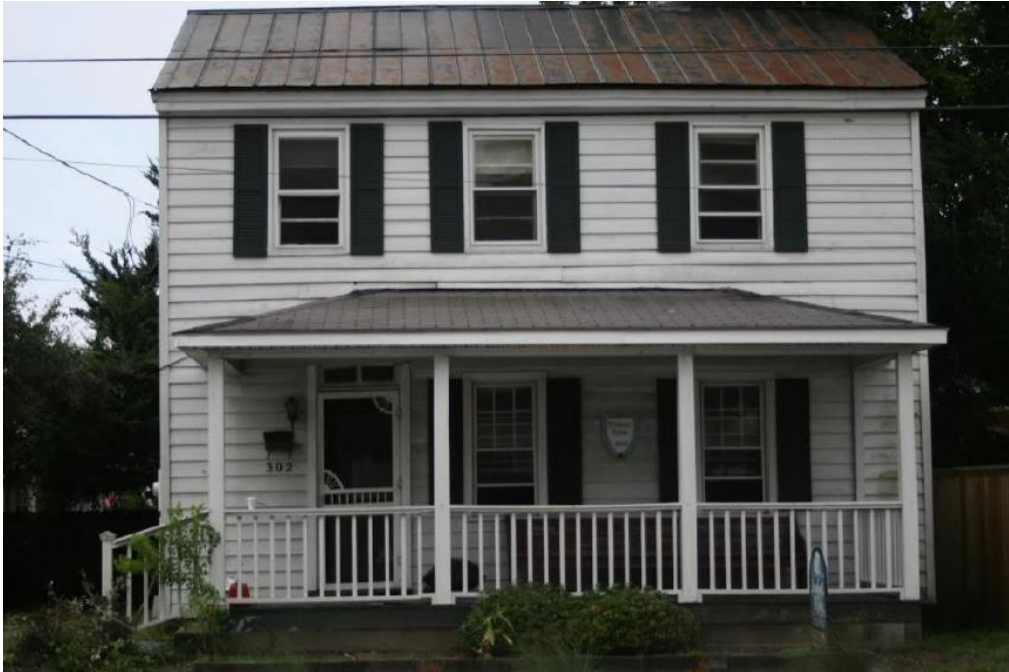
Front view of 302 Cedar Street
