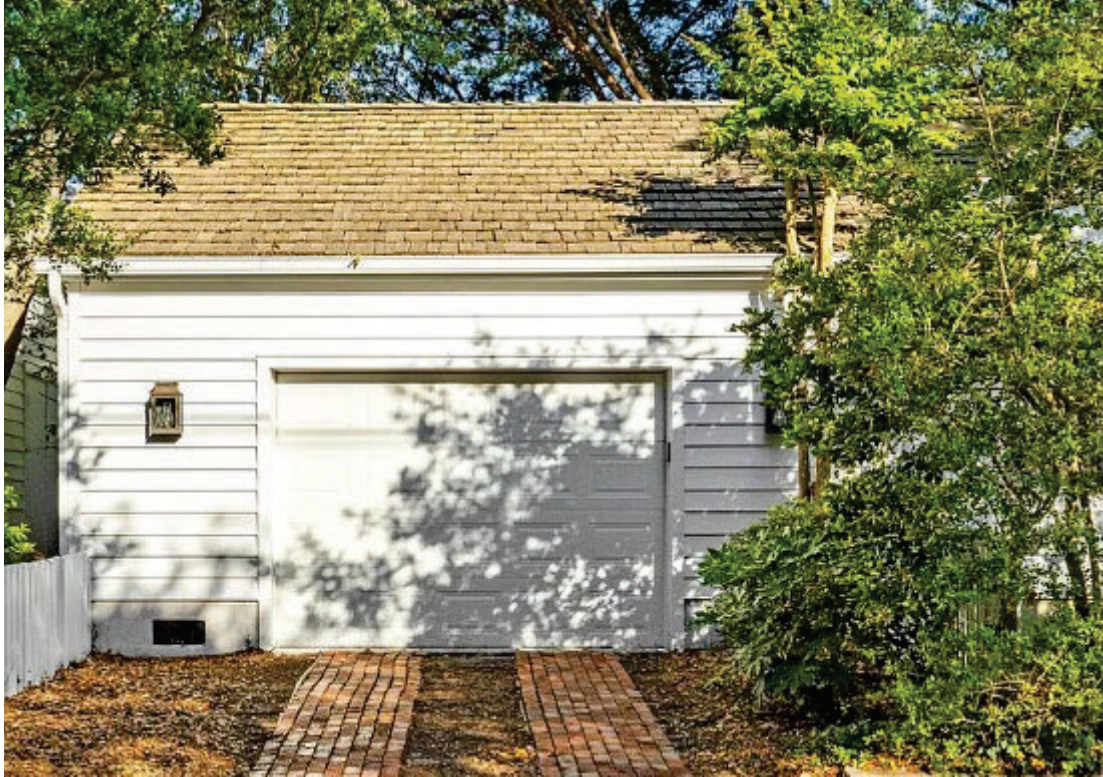
West Side of Garage Roof attached to Guest House
