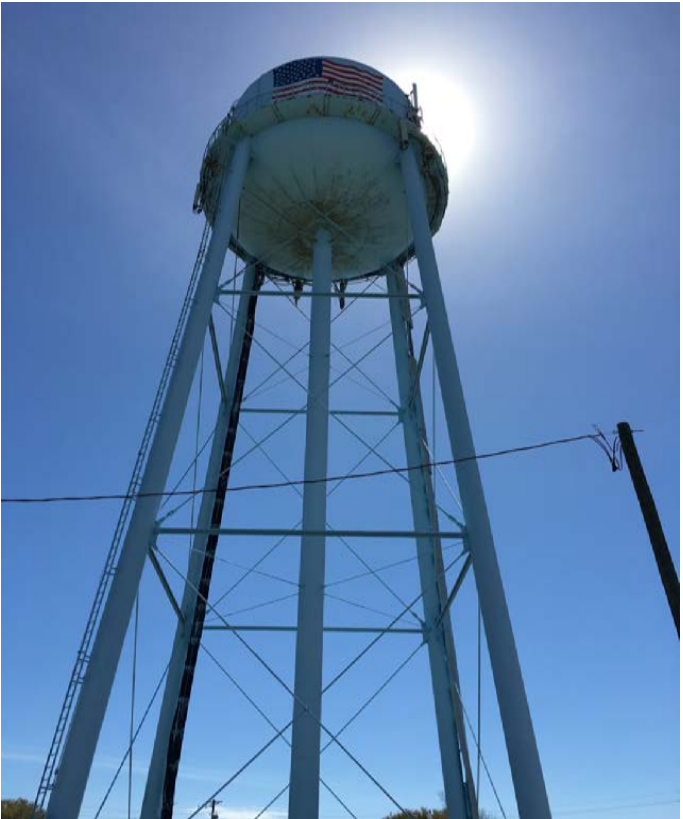
Beaufort Water Tower
