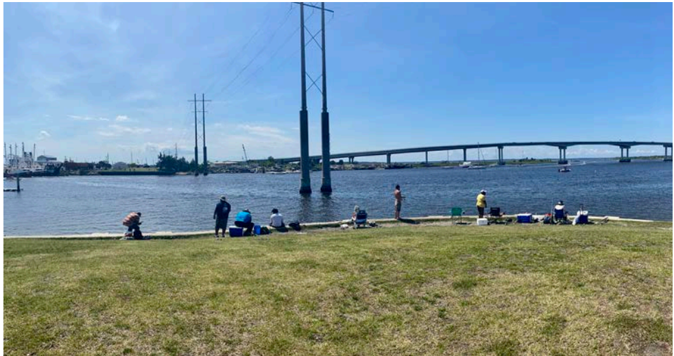
Gallants Channel Bridge
