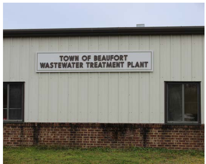
Town Wastewater Treatment Plant
