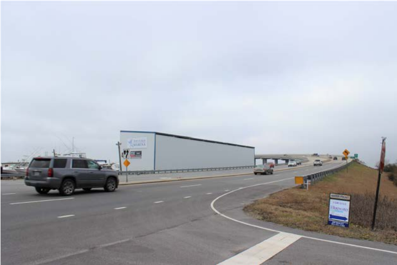
Highway 70 bridge over Gallant's Channel
