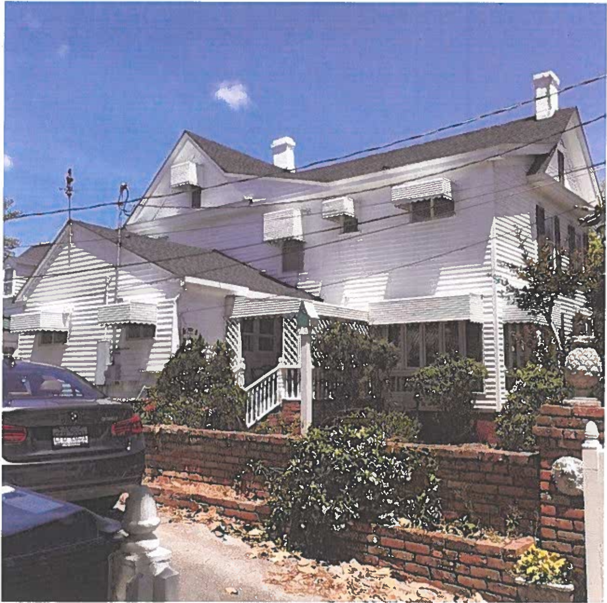
Former Porch enclosure
