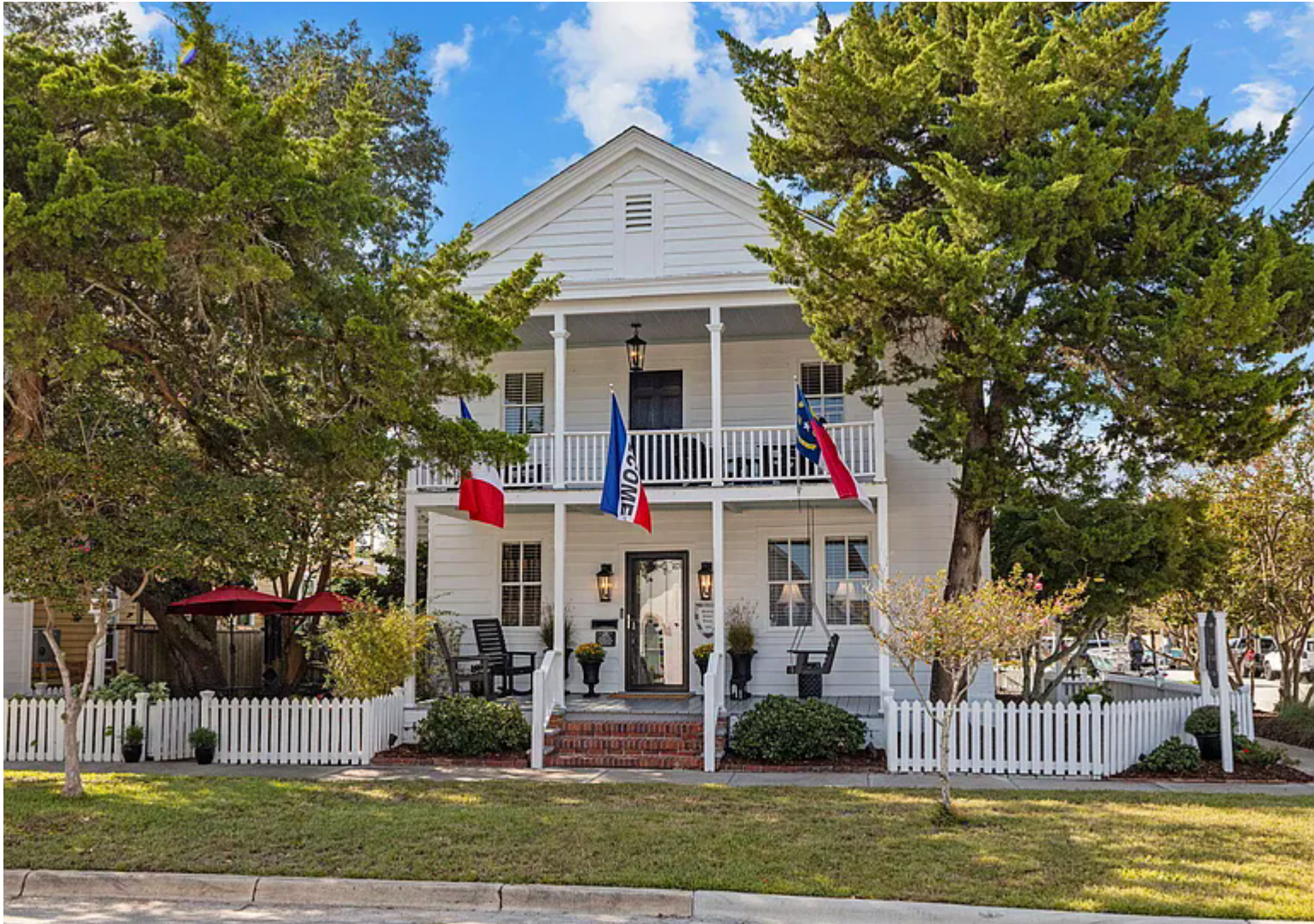
FRONT OF HOME (TURNER STREET)
