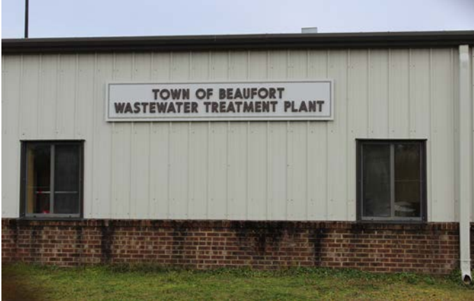
Town of Beaufort Wastewater Treatment Plant
