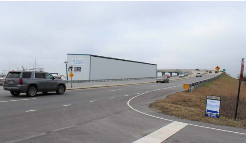
Highway 70 bridge over Gallant's Channel
