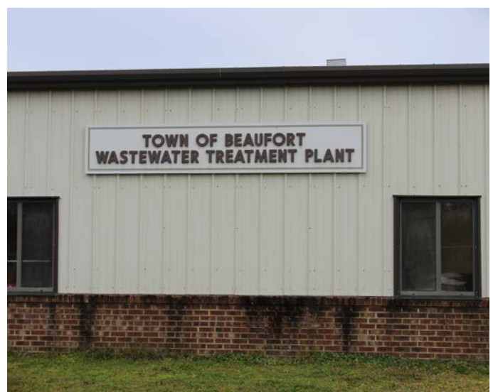
Town Wastewater Treatment Plant
