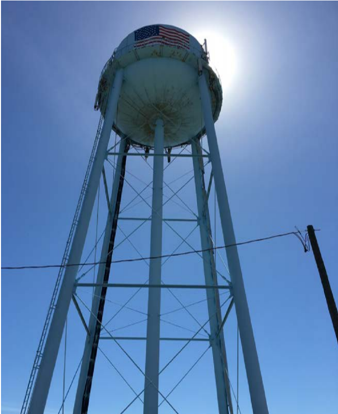
Beaufort Water Tower
