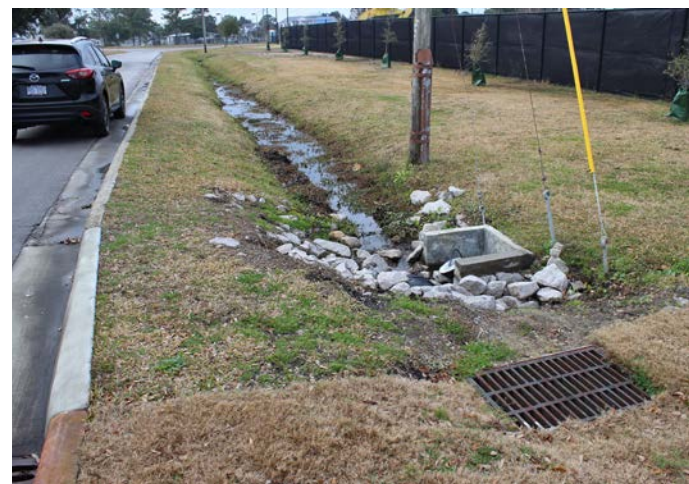
Stormwater drainage area
