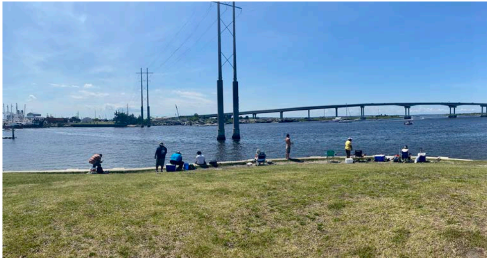
Gallants Channel Bridge
