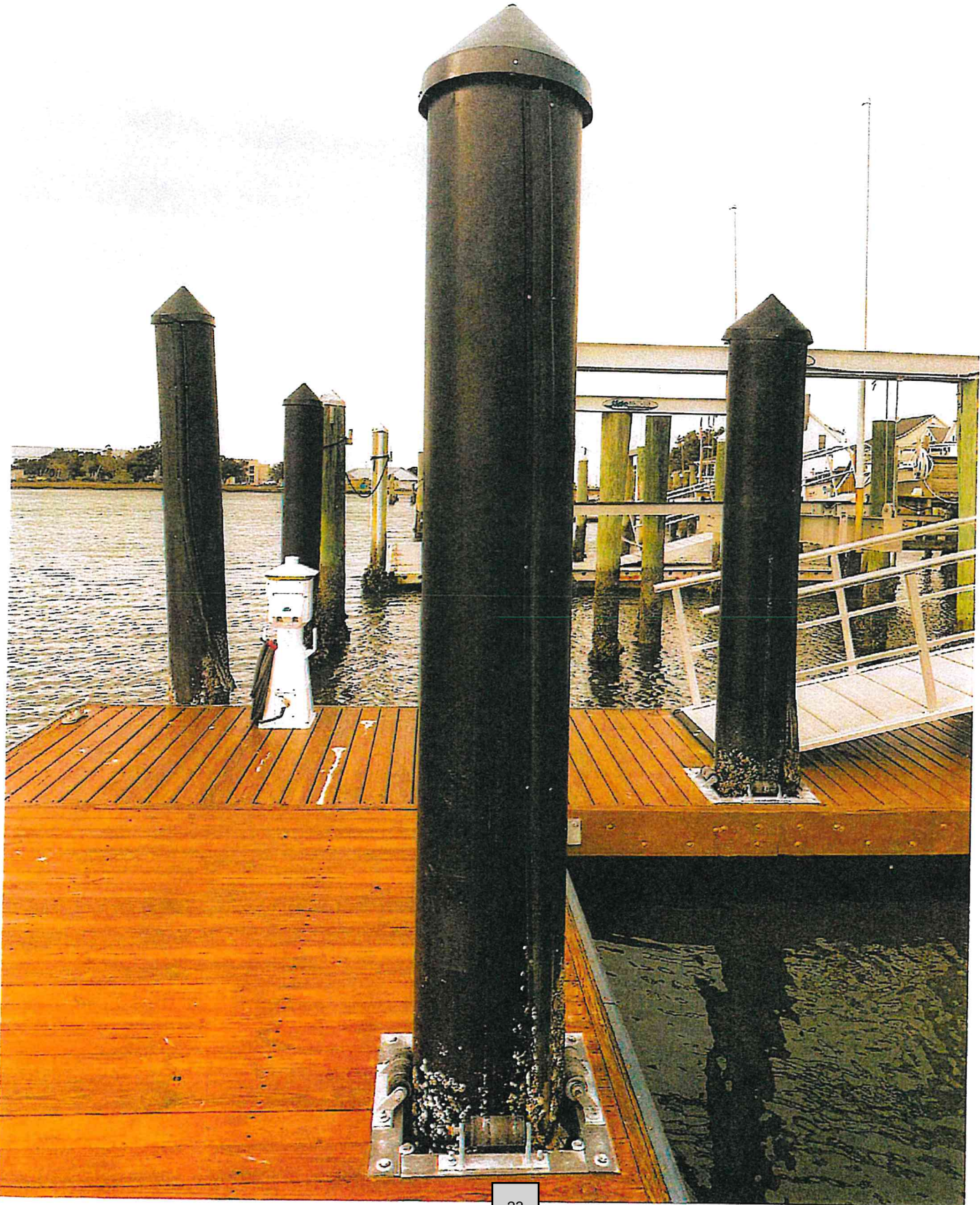
218 Front Street Proposed 12" Diameter Black HDPE Pile Sleeves with Black HDPE Pile Caps
