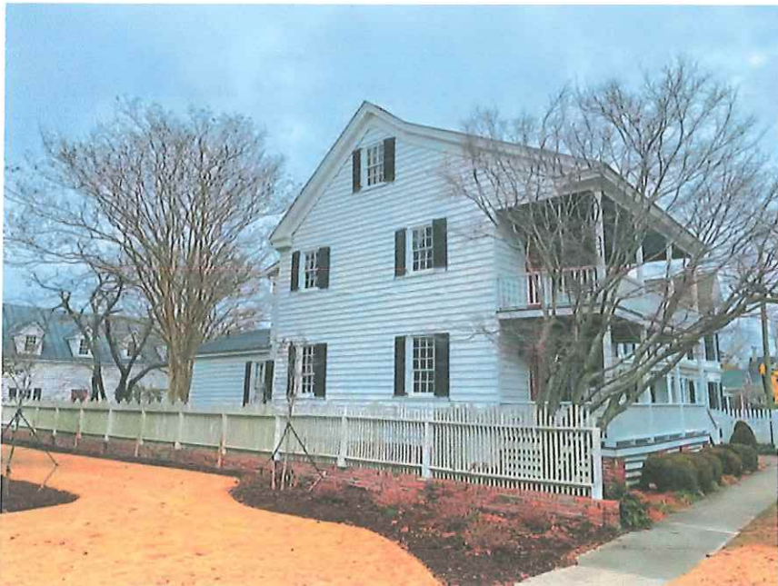
(C) South West View of House (winter) - 2022
