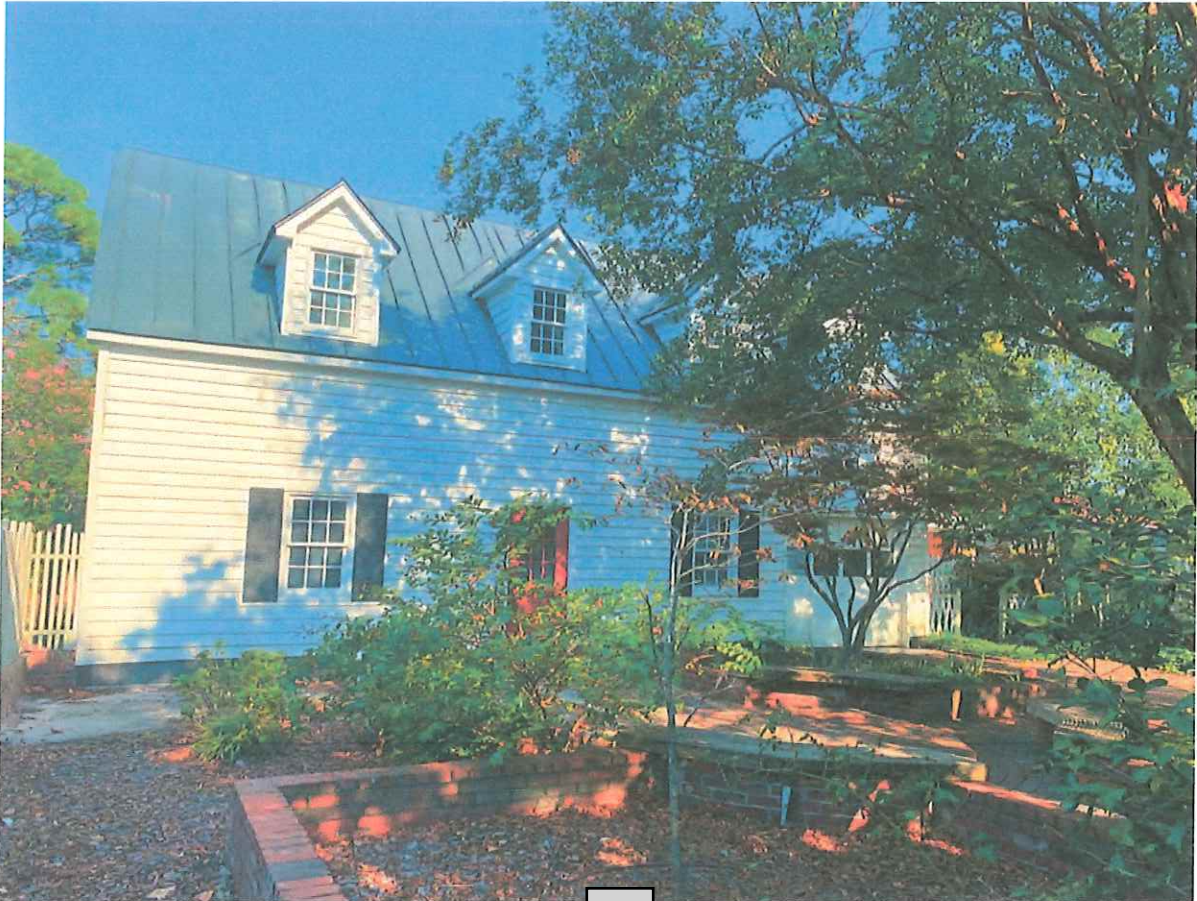
Brick Courtyard between Existing House 19 Existing Accessory Structure
