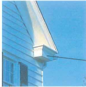
Gable end return features heavy frieze boards with small crown. Crown on fascia, with flat return
