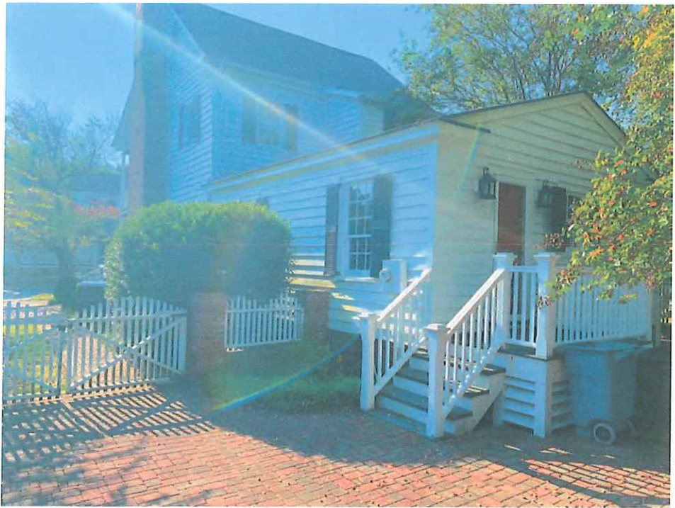
View of Existing Single Story Rear Additions to House
