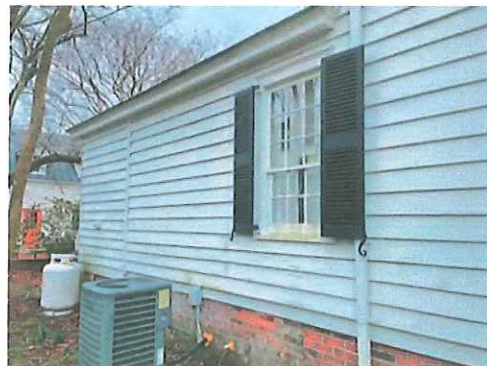
Vertical trim mid wall denotes another addition or absorption.
