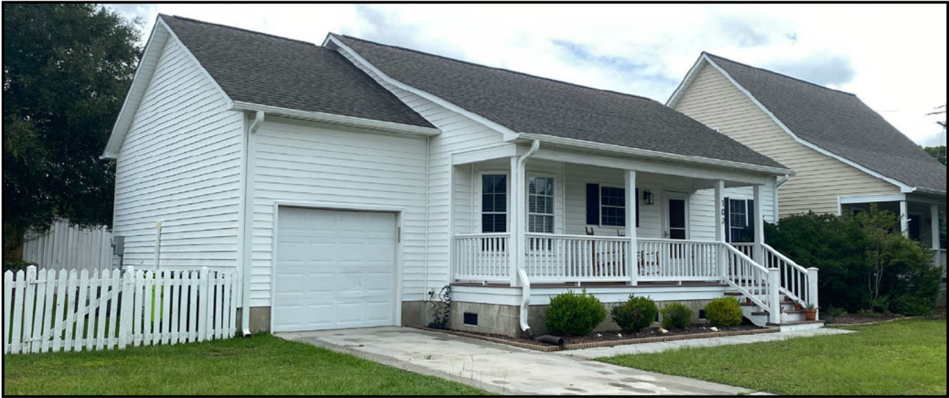
102 BEAUFORT WALK. FRONT CORNER
