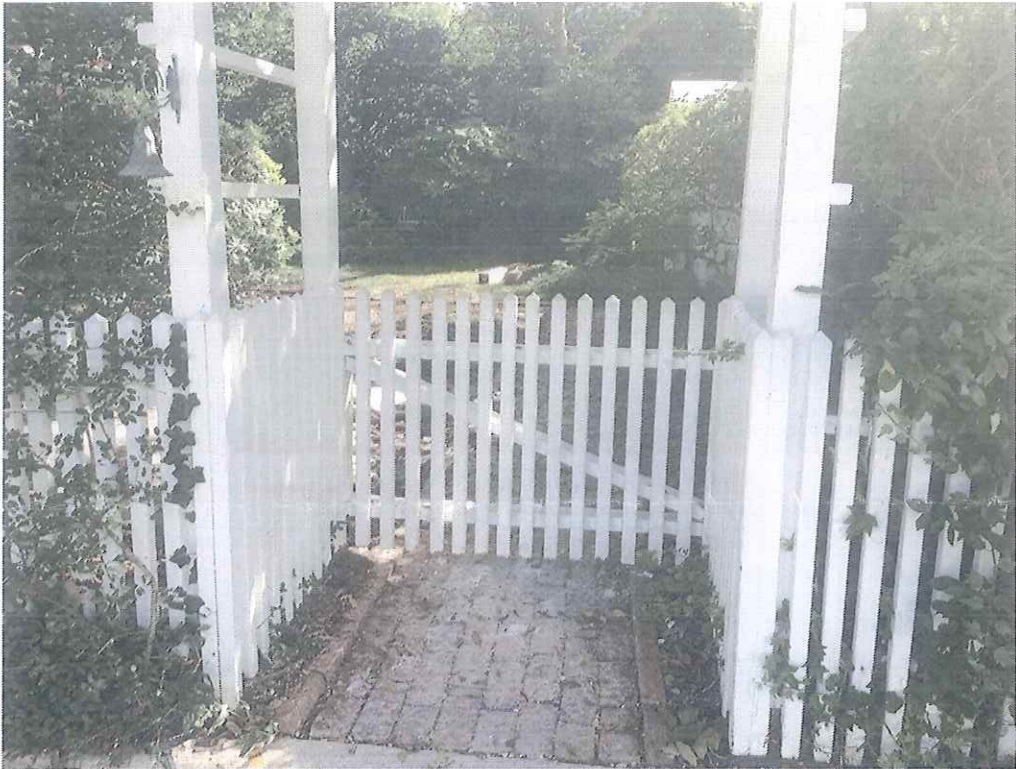
Picture to the left is of the existing fence located at 201 Front Street, Beaufort.
