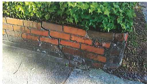
Adjacent neighbors brick wall for reference 110 Orange Street, Beaufort, NC
