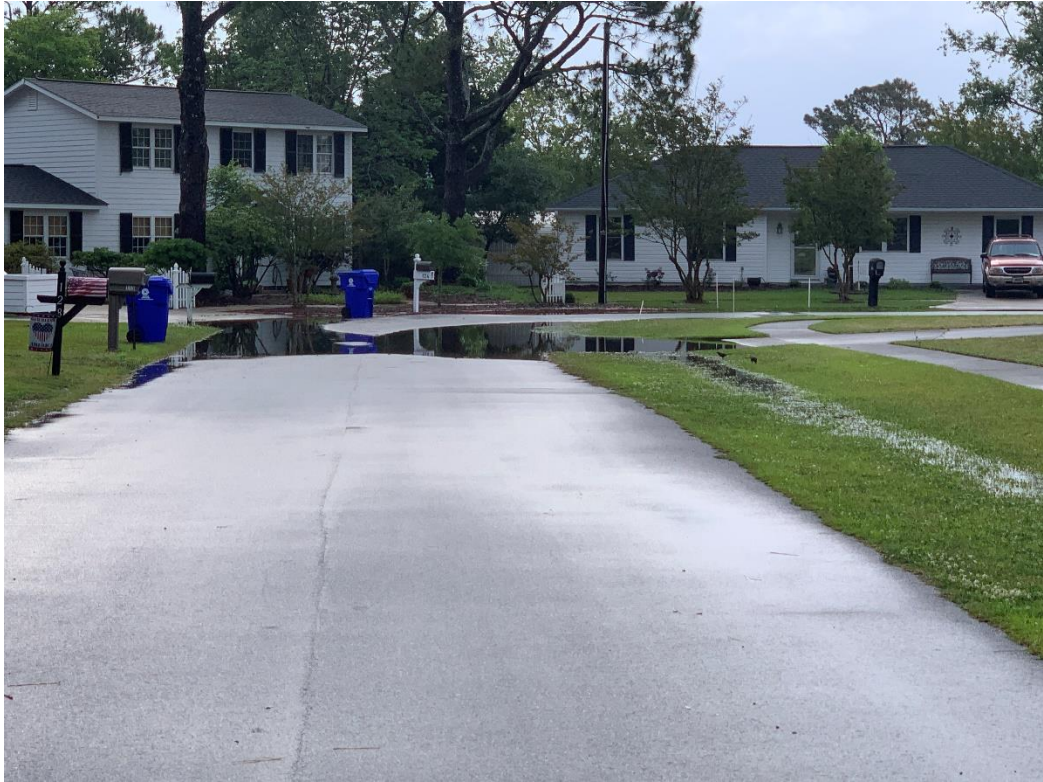
Charles Street road flooded after a normal rainfall (5/22/2020).
