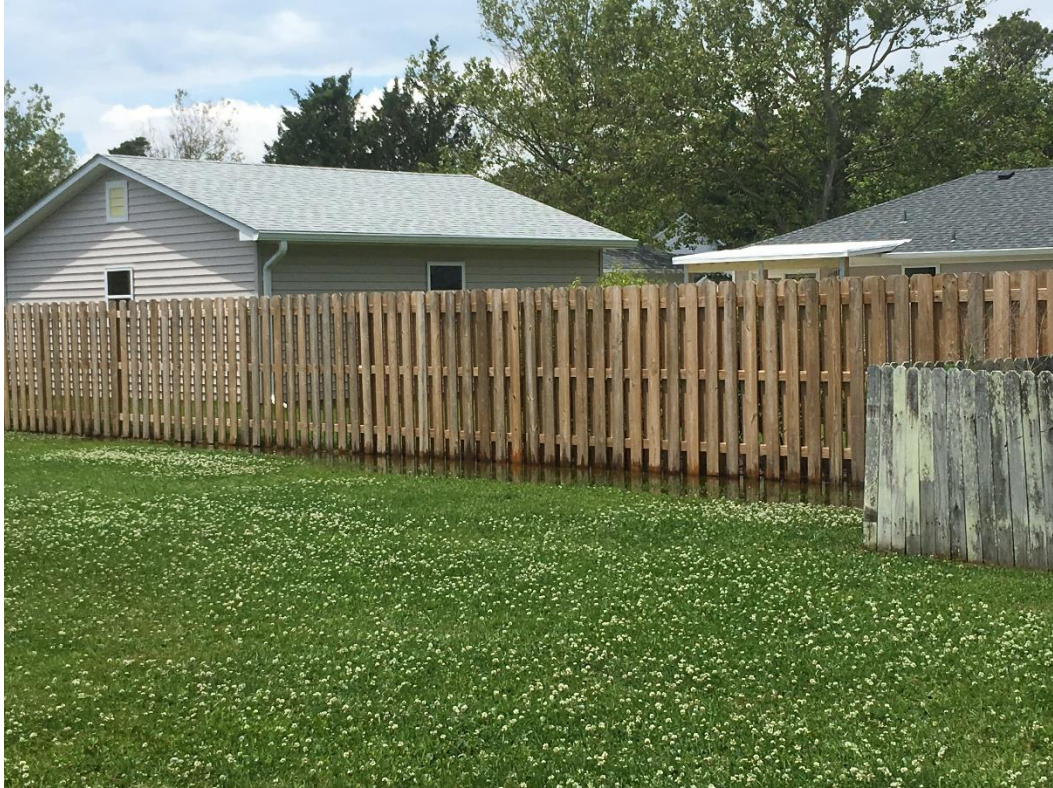
Backyard of Charles Street property flooded after a normal rainfall (5/22/2020).
