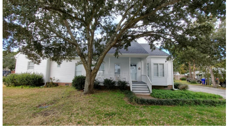
Existing East Elevation (Street)
