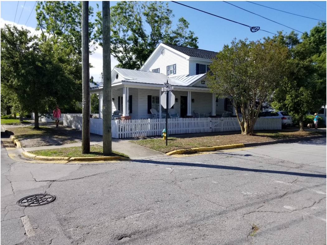
216 ORANGE STREET (ACROSS ORANGE STREET FROM SITE)
