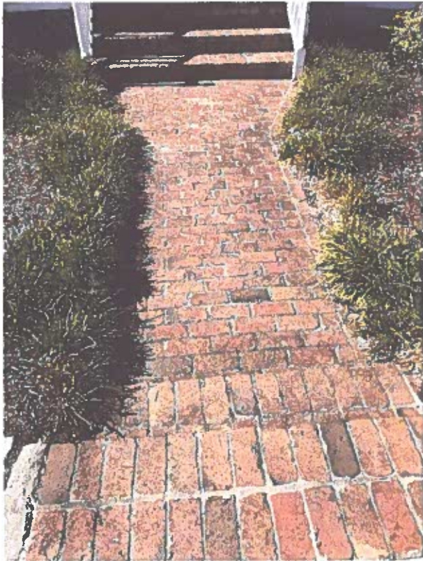
Steps and walk at 129 Craven (brick used for steps and walk)
