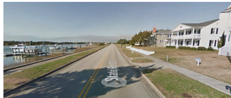
Front Street East of Hill Street
