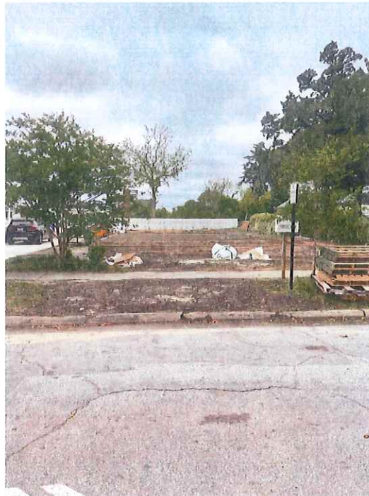
308 Ann St – First Baptist Church, foundation directly adjacent to the west
