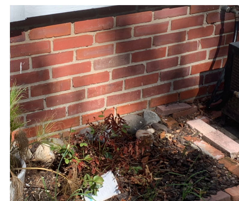
EXISTING BRICK FOUNDATION
