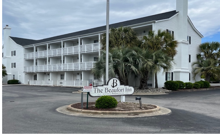
North Elevation View of Beaufort Inn
