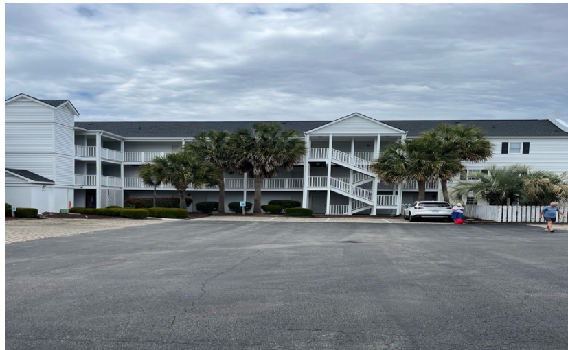
South Elevation View of Beaufort Inn
