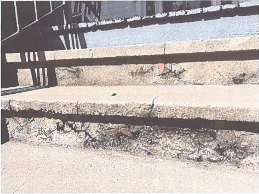
Steps were created with cement over brick
