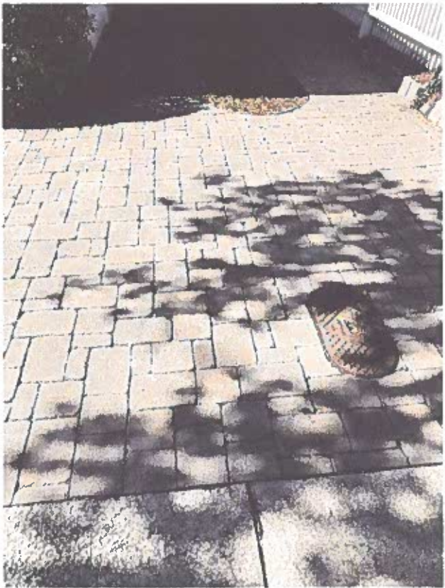
Path and drive at 131 Craven
