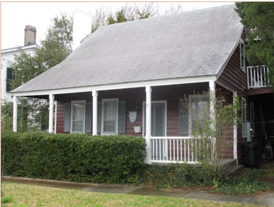
The typical porch of a coastal cottage is created by the roof extension on the front façade, such as in this 18 th century house on Ann Street.
