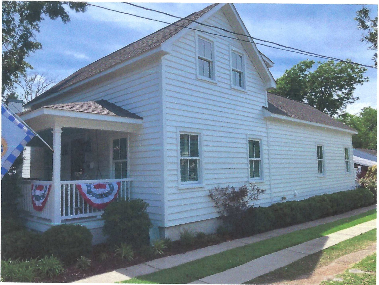
Current View of House Front and Side
