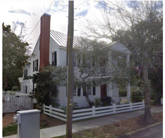
118 Moore Galvanized Tin Roof
