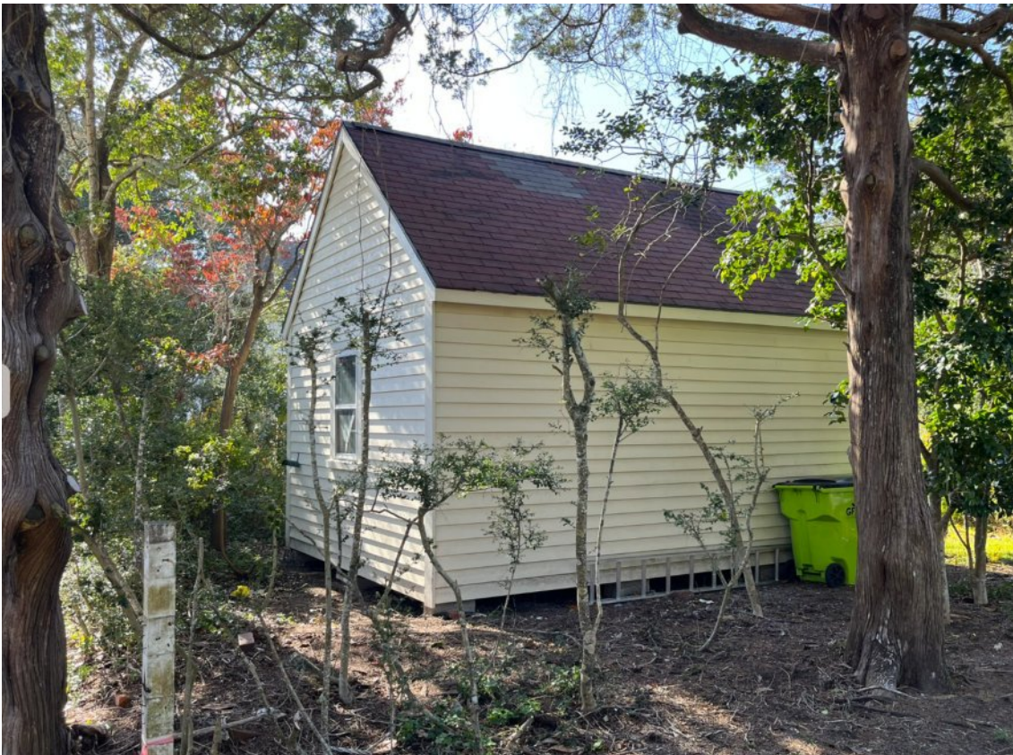
Accessory structure rear corner viewed from adjacent cemetery
