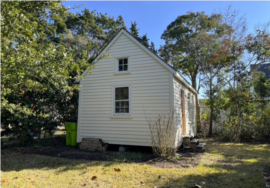
Accessory structure close up viewed from backyard - Moore Street side
