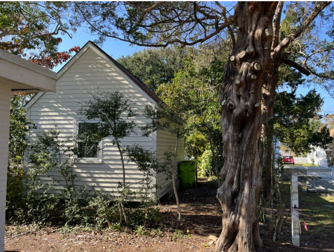
Rear corner viewed from cemetery looking towards Moore Street
