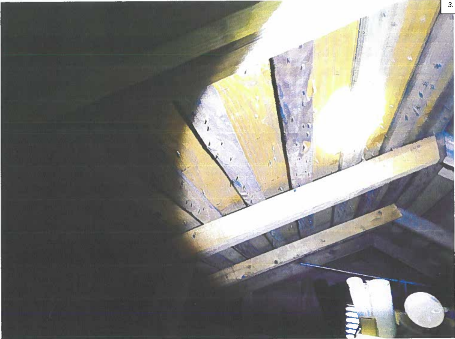
Additional scabbed on rafters & plywood sheathing
