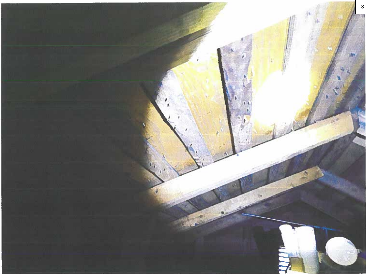
Additional scabbed on rafters & plywood sheathing
