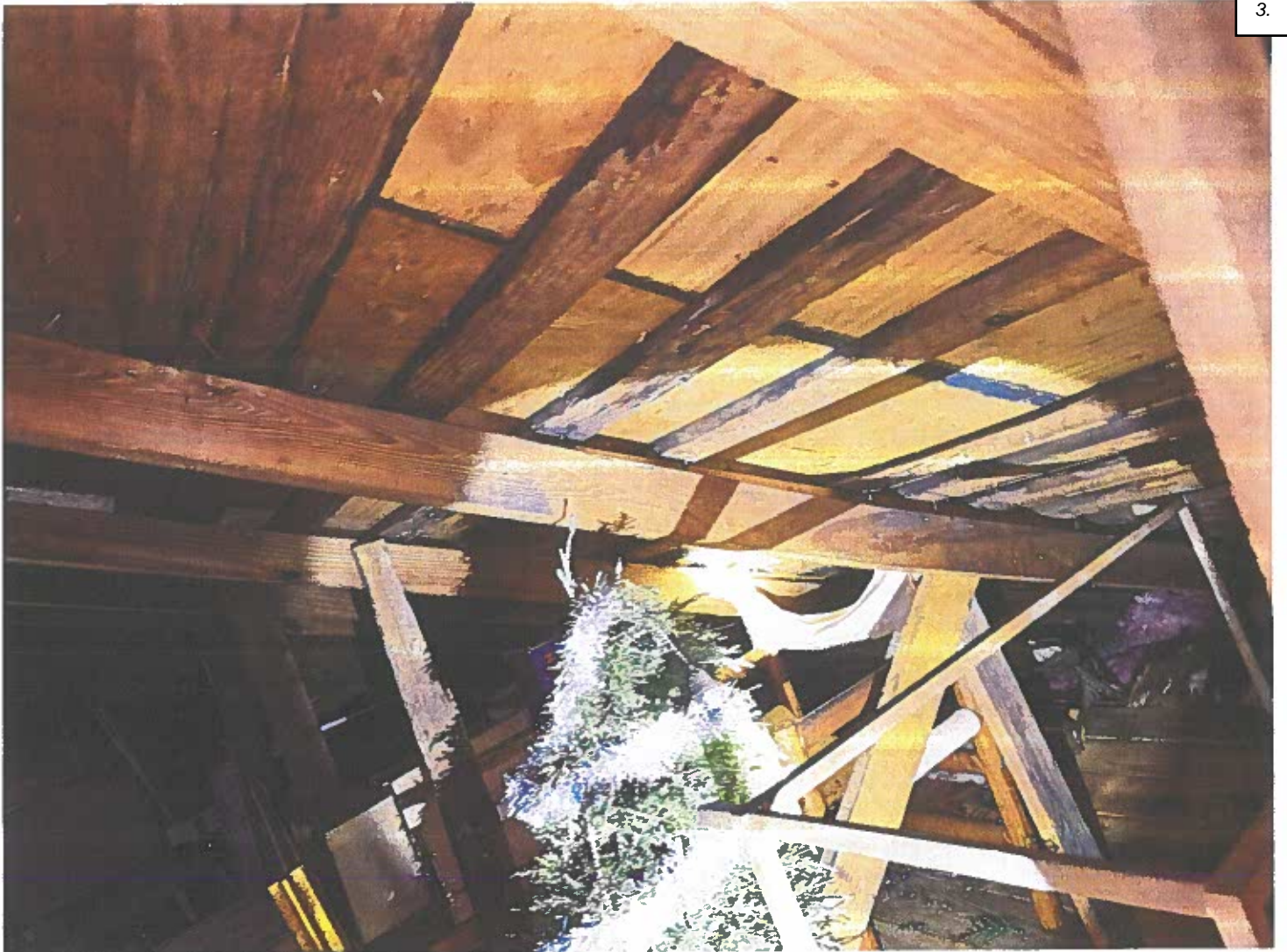
Additional scabbed on rafters & plywood sheathing
