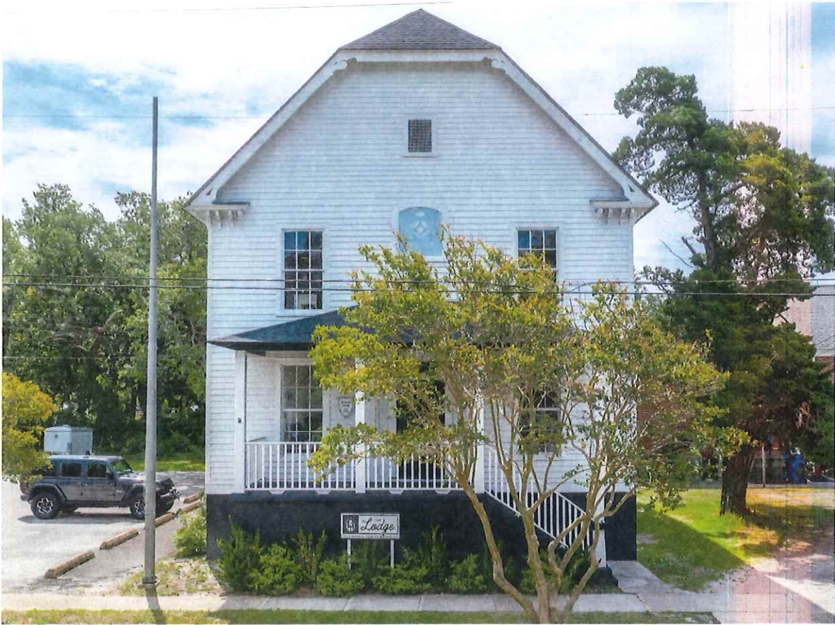
View of West facade. Existing to remain. Circulation towers to be added to the North facade will match existing conditions and be an extension of the original structure. Existing Crepe Myrtle to be removed. Two parallel parking spots or "loading zone" spots proposed on Turner Street.
