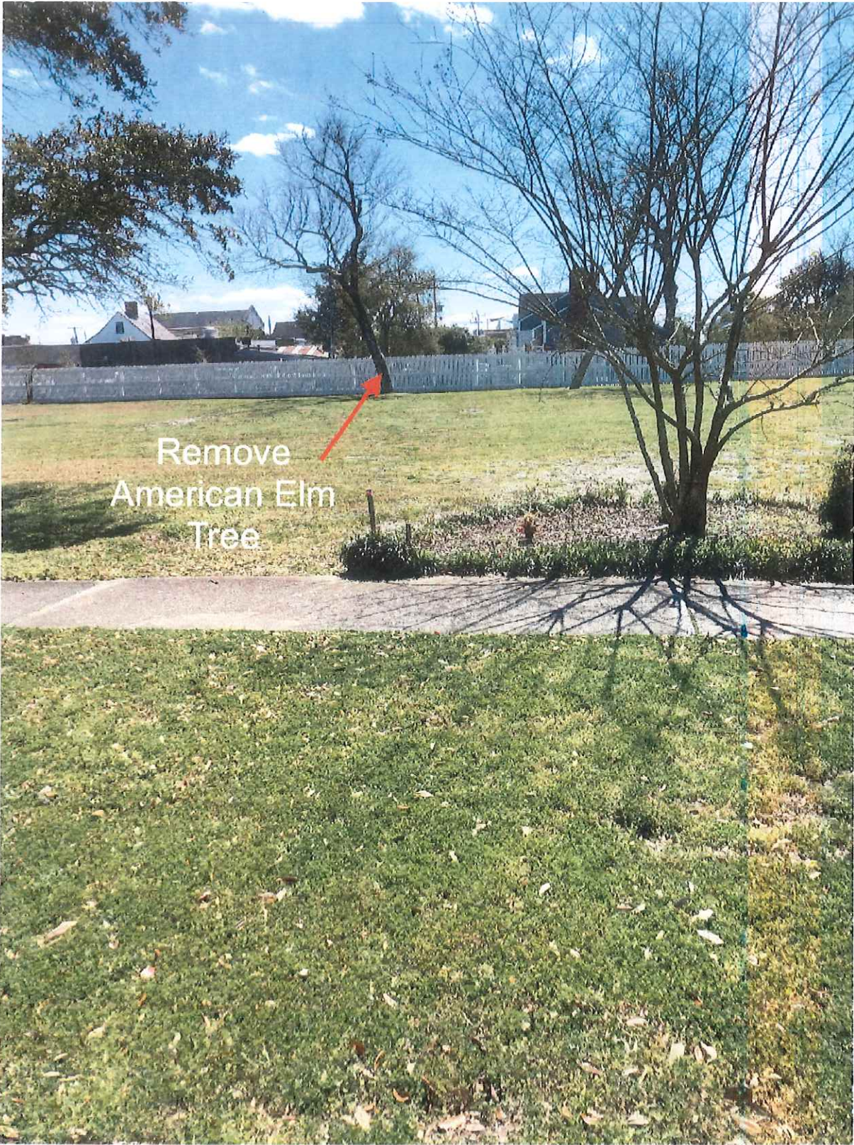
2. American Elm Tree is the only tree on 310 Ann property in this photo and is to be removed because it is within excavation footprint.
