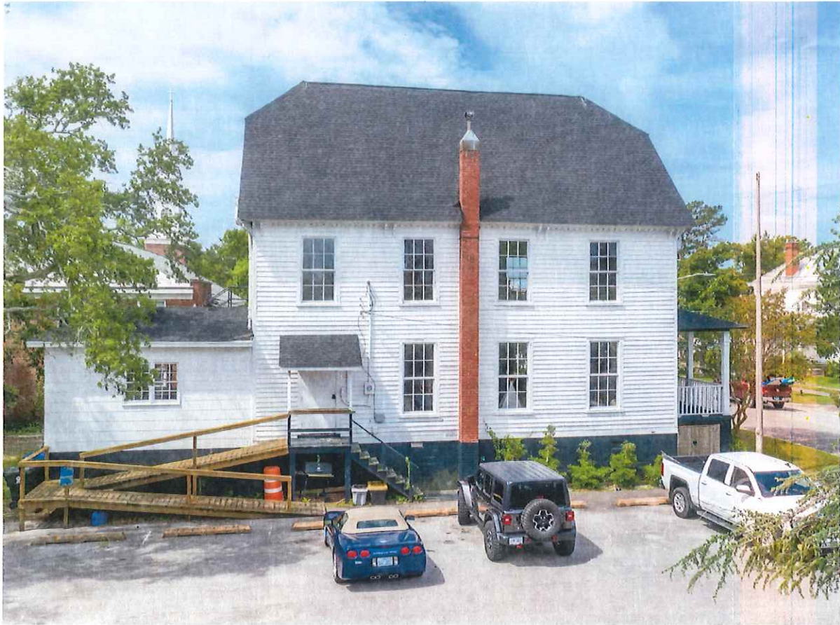
View of North facade. Proposed new construction to extend approximately 64 feet to the East and will match existing structure. Chimney, porch stoop, stairs, and ramp will be removed to accommodate 3 circulation towers for elevator and stair access. Parking lot will be reworked and expanded to include more parking and handicap accessible spots.
