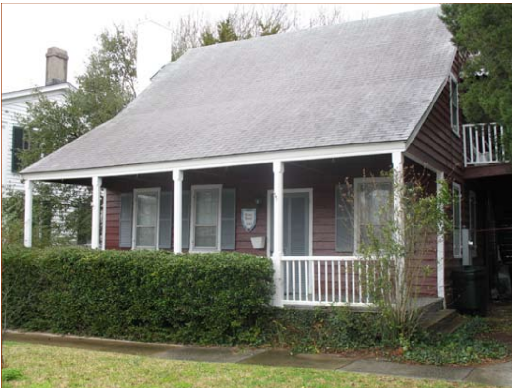
The typical porch of a coastal cottage is created by the roof extension on the front façade, such as in this 18 th century house on Ann Street.
