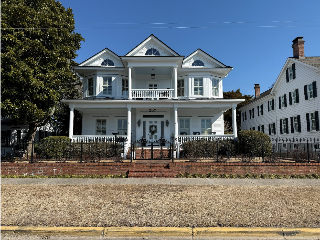
207 Front Street – Existing masonry wall and elevated grade relative to sidewalk and street.
