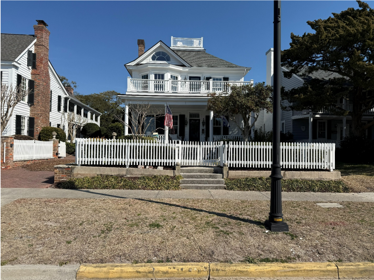
217 Front Street – Existing masonry wall and elevated grade relative to sidewalk and street.
