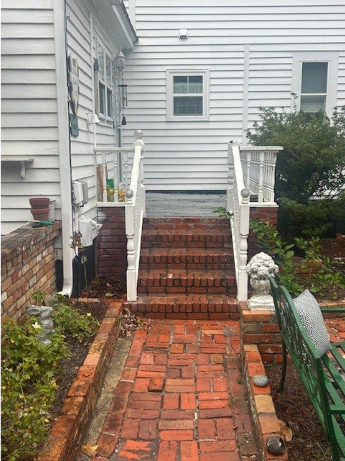
North Facing back porch
