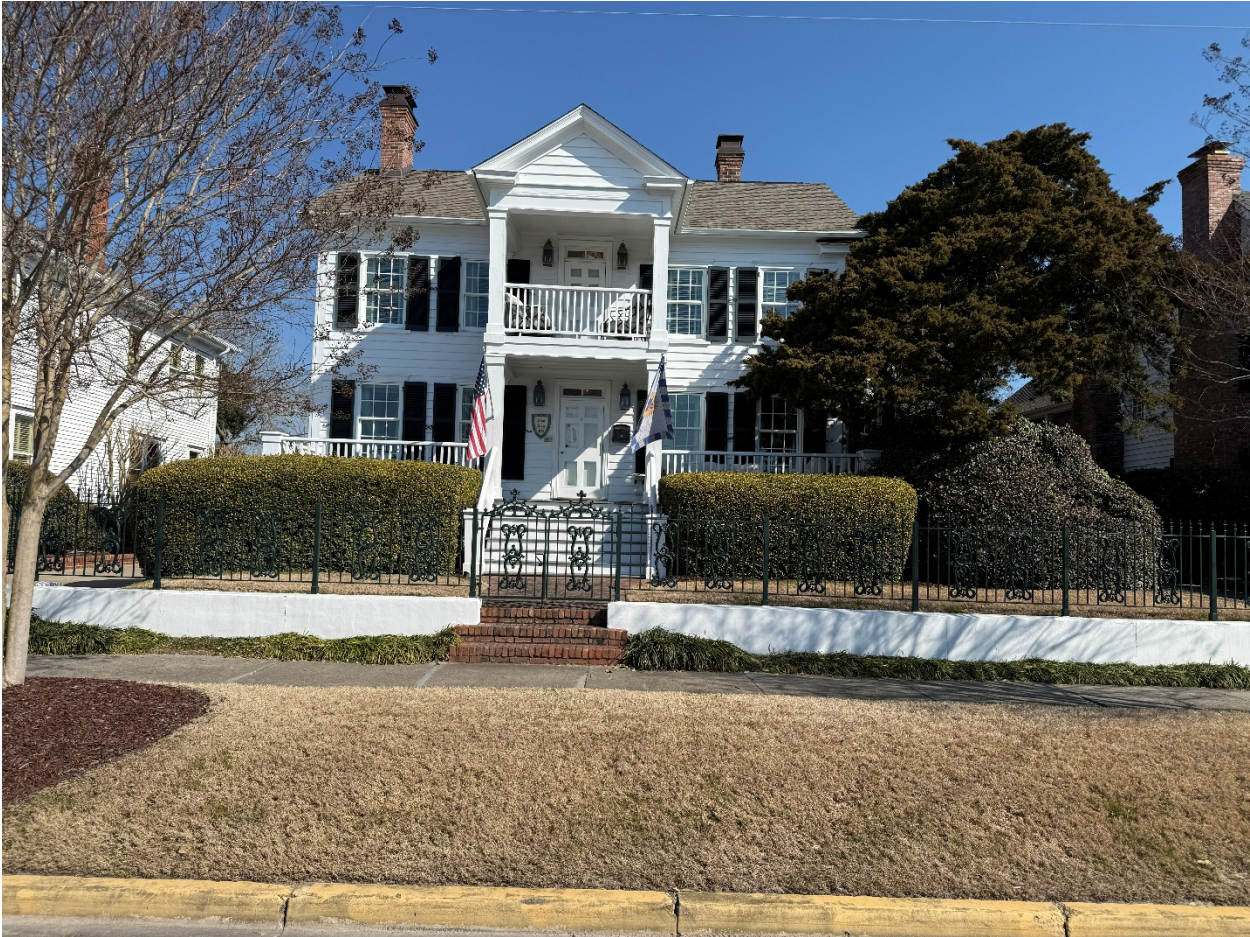
209 Front Street – Existing masonry wall and elevated grade relative to sidewalk and street.
