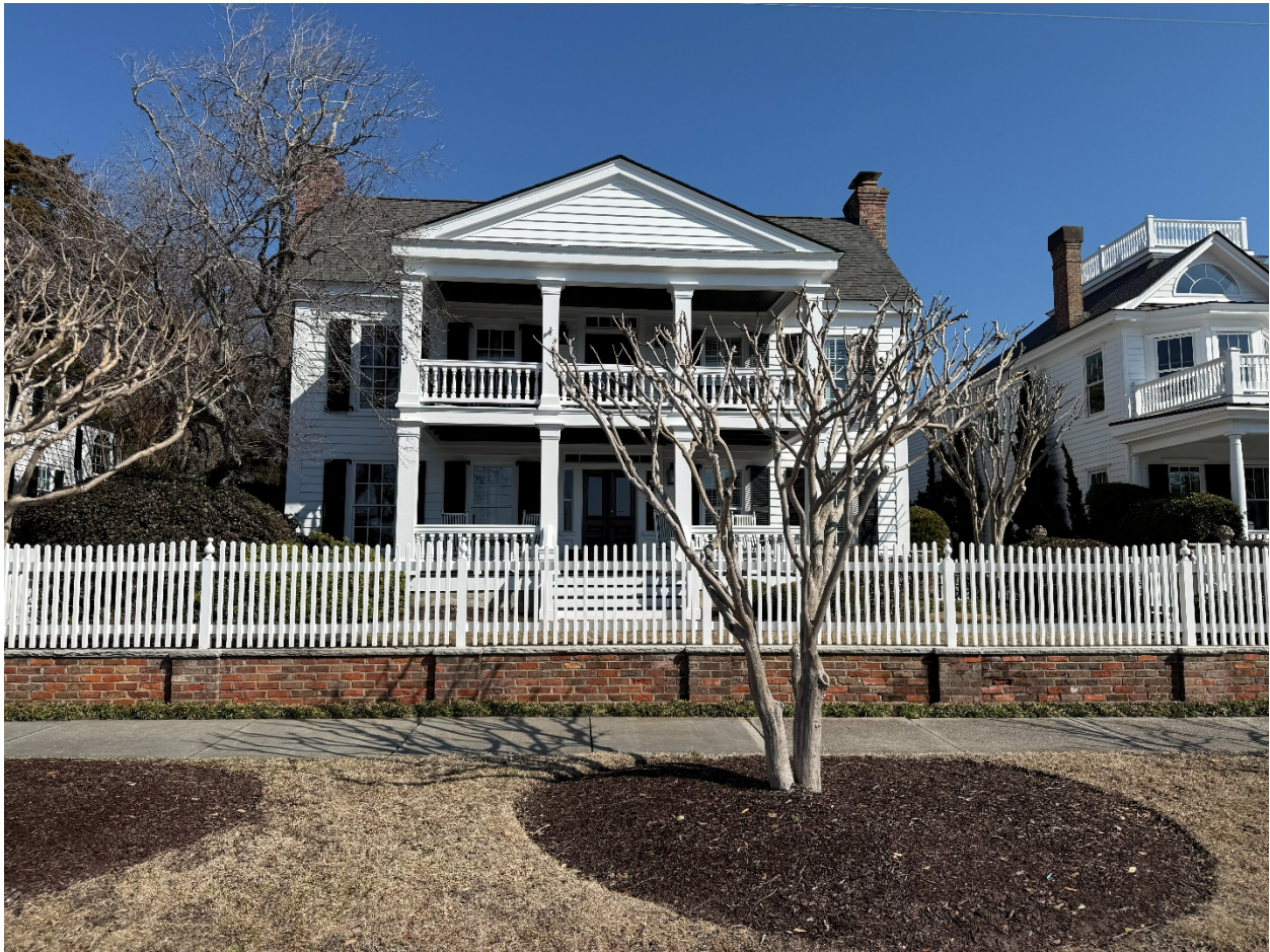
215 Front Street – Existing masonry wall and elevated grade relative to sidewalk and street.
