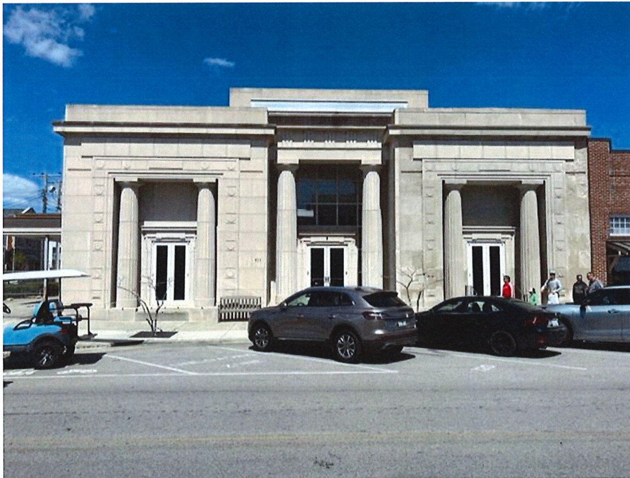
South elevation of the existing First Citizens Bank building to remain unchanged.
