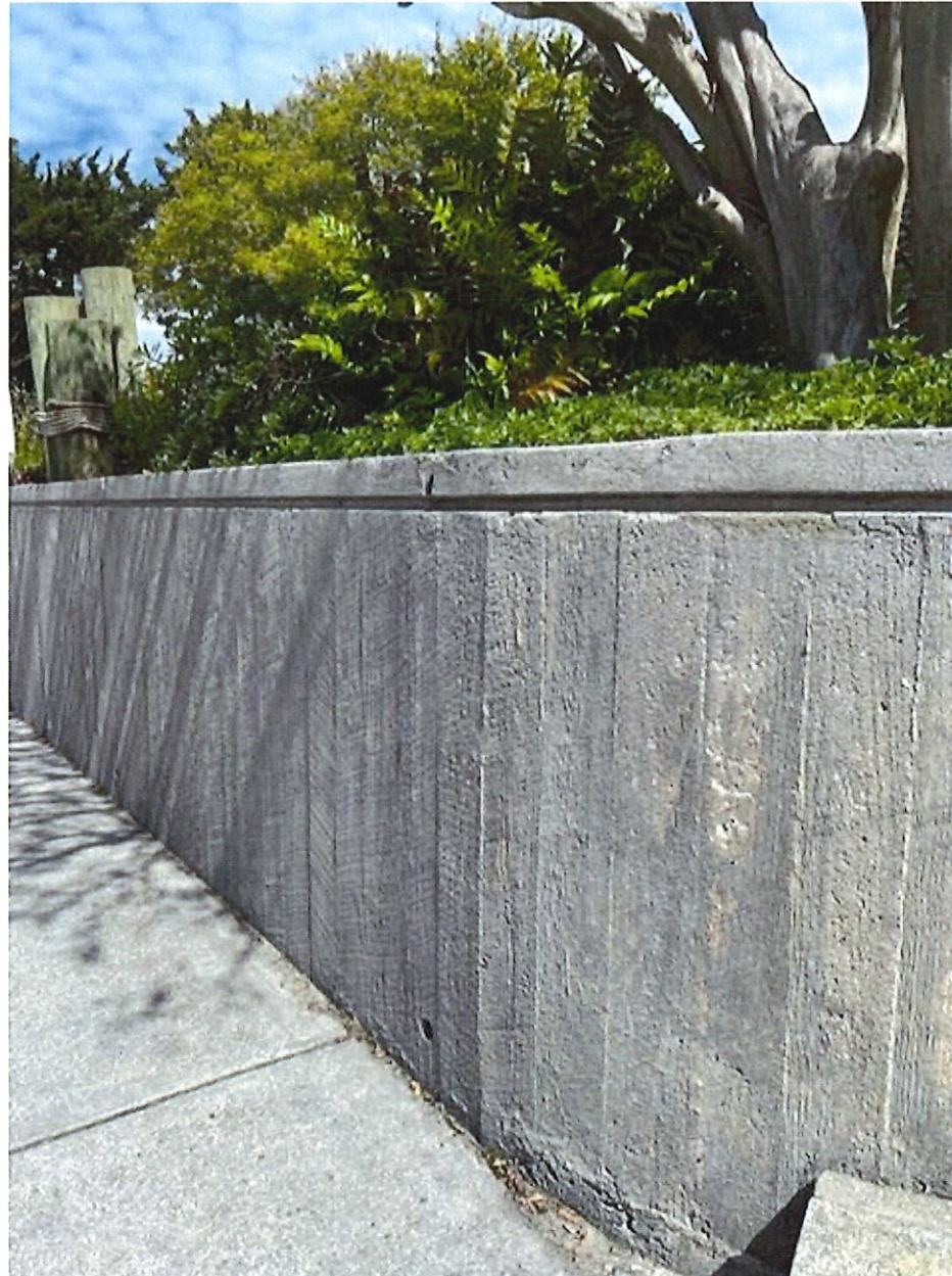
Poured in Place Concrete Wall. Option#2
