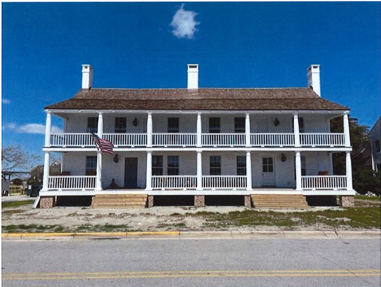
South Elevation of Duncan House where proposed “Paver walk”, and “Turf” will be in Town of Beaufort Right of Way.
