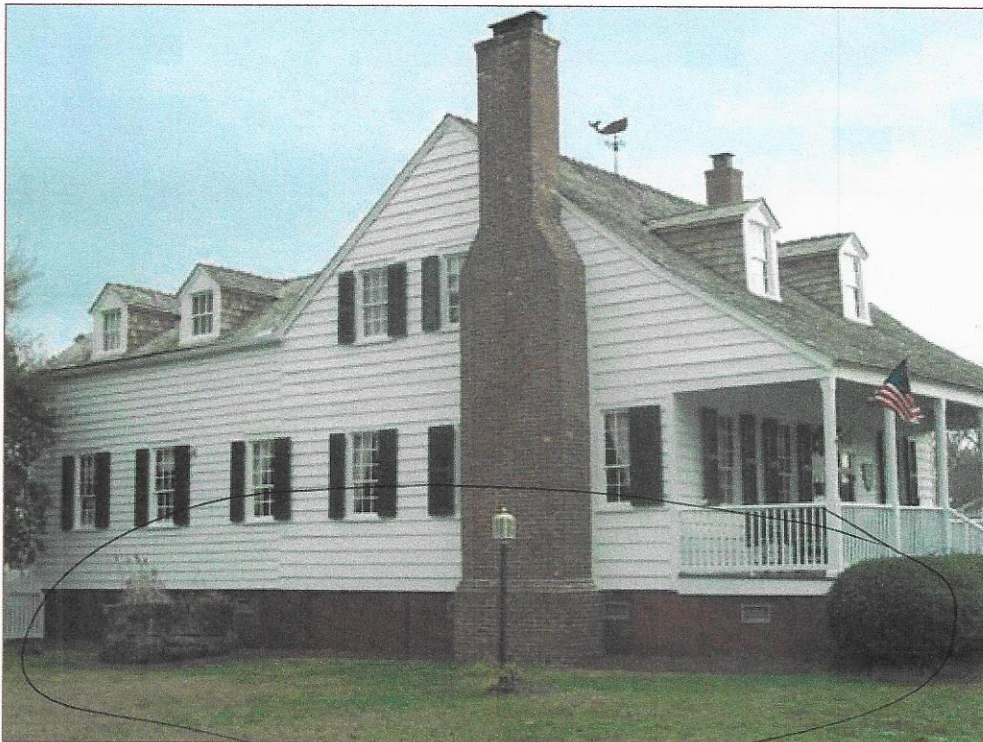
Federal Style; Mace House (c. 1831), 619 Ann Street
