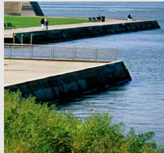
Open space can be flooded with little or no damage and provide recreation spaces when not flooded.
