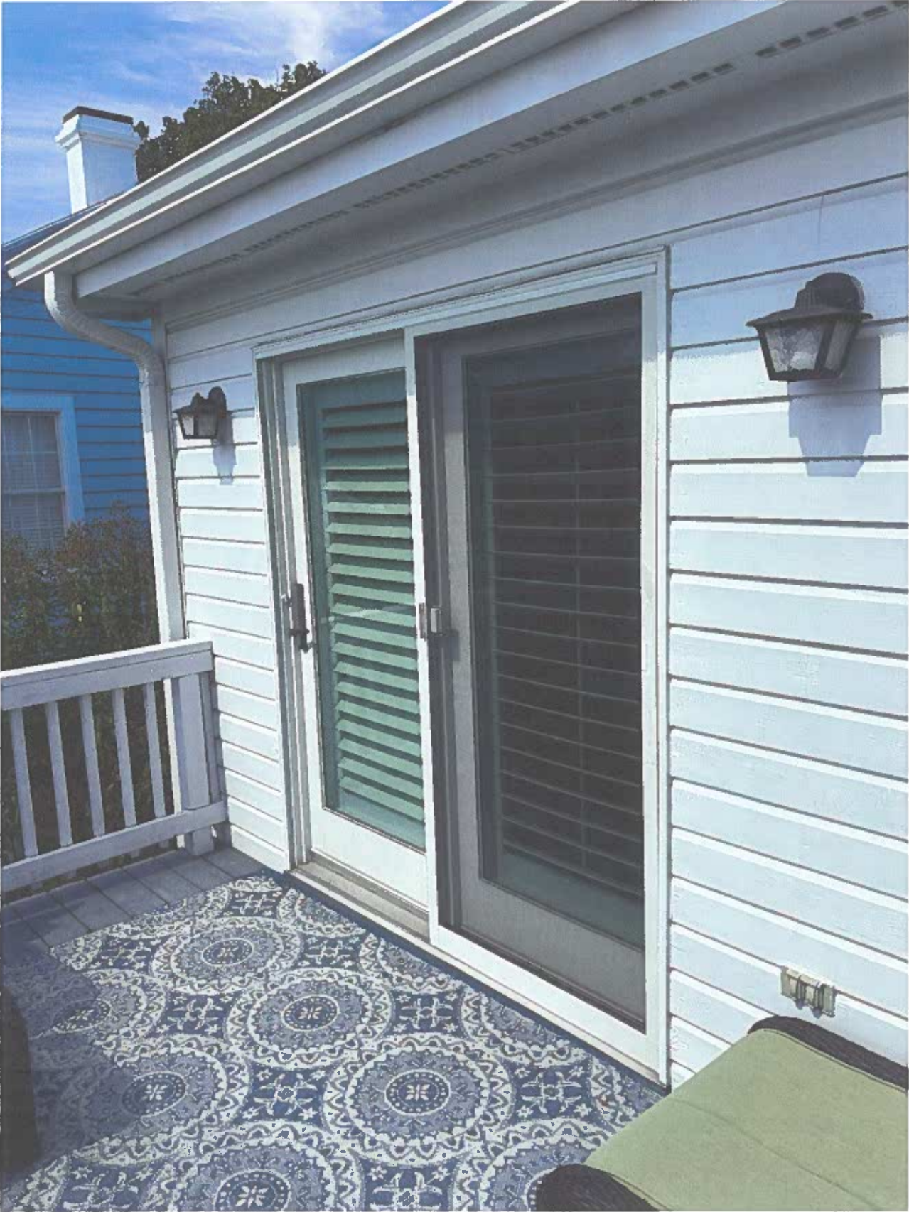
Photos of existing site, streetscape, and buildings impacted
