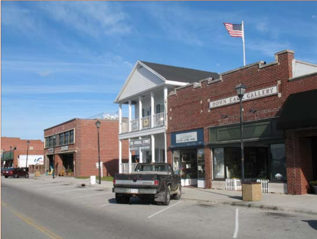
With few exceptions, commercial buildings along Front Street are one-and two-story masonry structures with brick façades, recessed entries, and large display windows.
