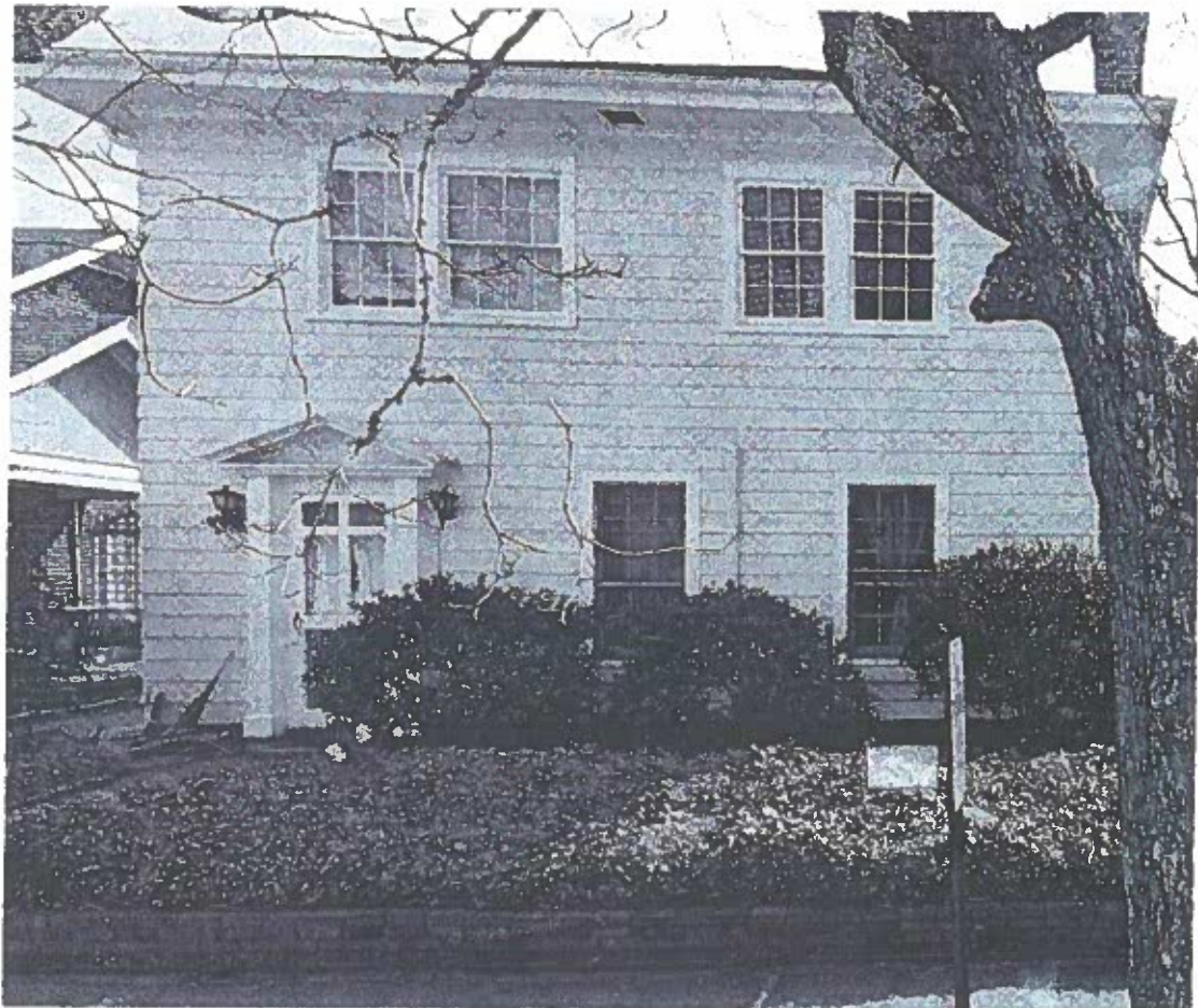
West Facing Front side of Home
