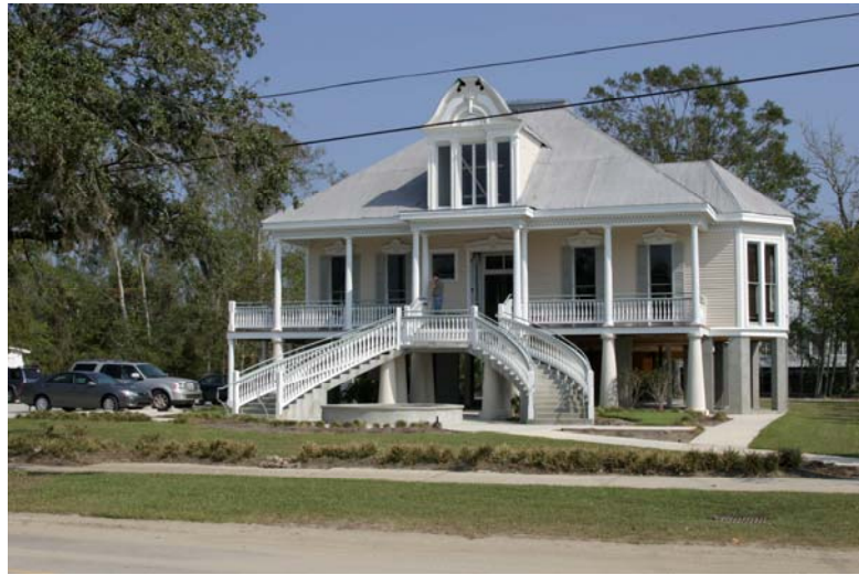
Elevation of a historic residence in Mandeville, Louisiana
