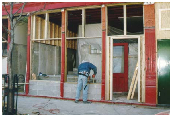
Floodproofing the vestibule of a storefront
