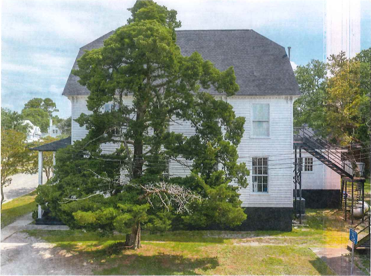
View of South facade. Original structure to remain. Building to extend approximately 64 feet to the east and match existing structure. Stairs at the rear to be removed, utility equipment to be relocated.
