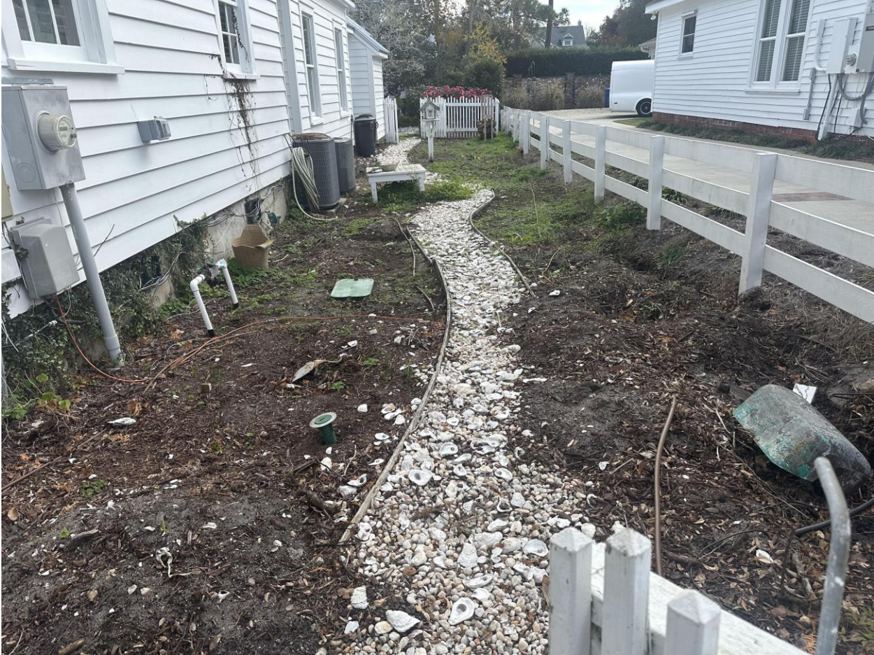
Right side landscaping install
